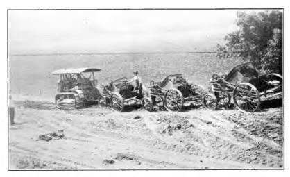
Fig. 1. Fulton County tractor and self-loading wheel scrapers grading a township road.
