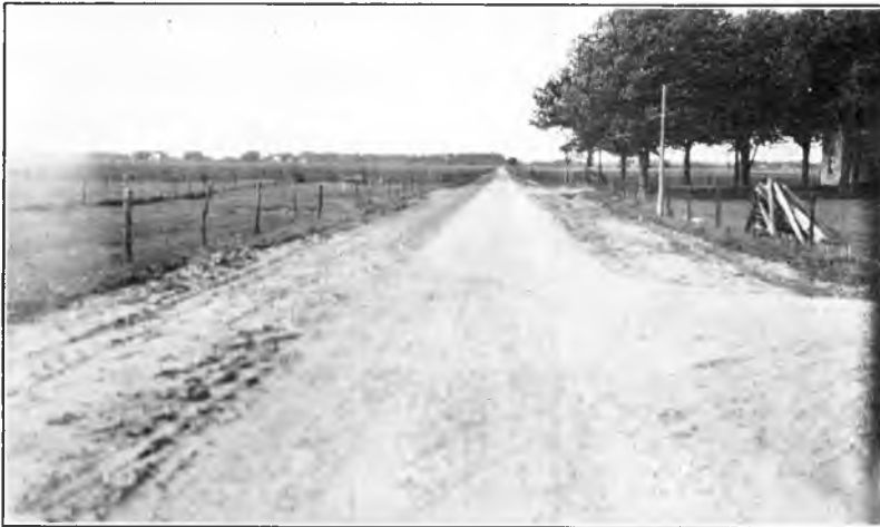
Fig. 1. Crusher-run stone road 10 inches thick, all passing one-inch circular screen.
