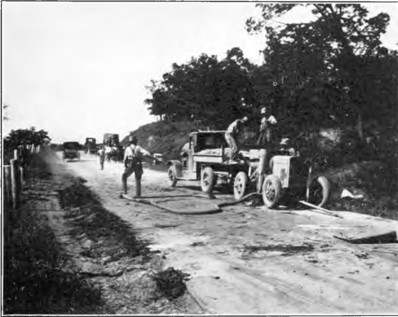
Fig. 10. Raising a section of pavement with Poulter mud pump.
