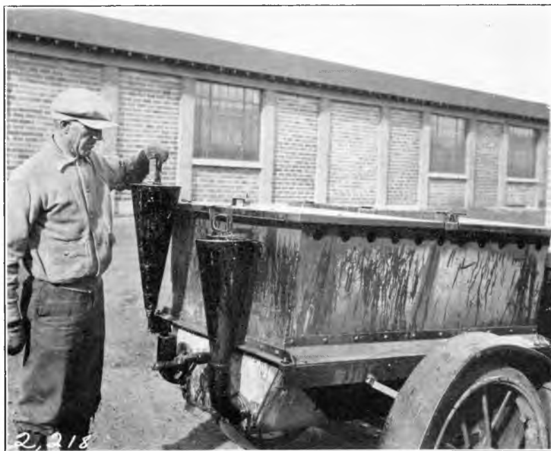
Fig. 7. Bituminous pouring pot heater attached to bituminous kettle.
