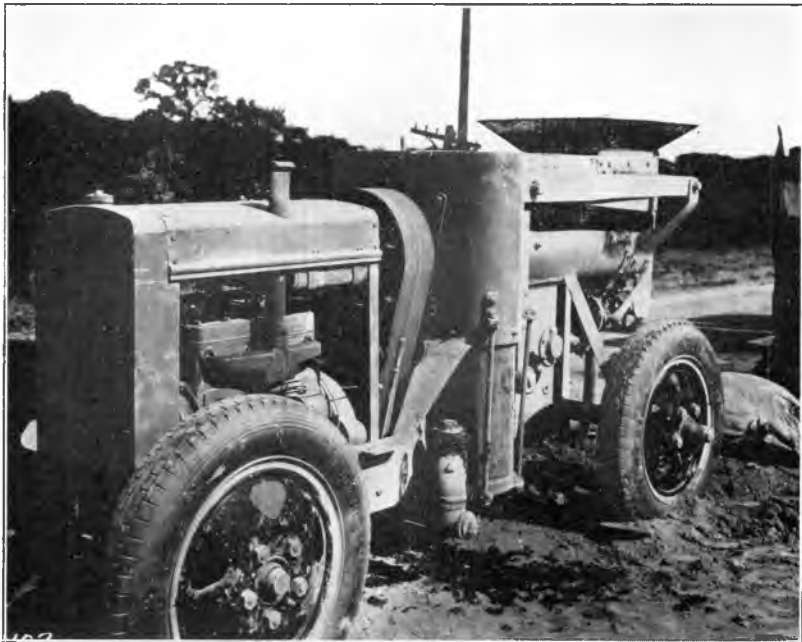
Fig. 8. The Poulter mud pump for raising settled pavement slabs.
