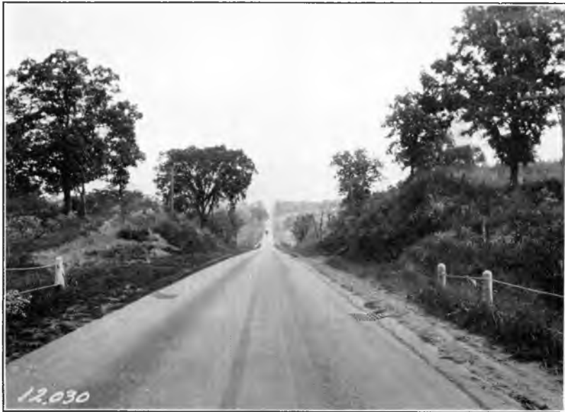
Fig. 1. Sloping curb section used on hills.
