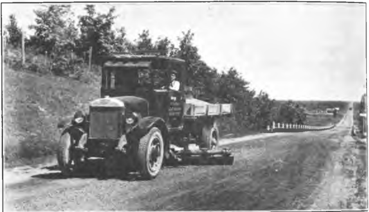
Fig. 1. Spring Blade attached to truck.
