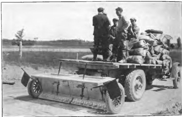
Fig. 2. Equipment used in applying Calcium Chloride on Gravel Road.
