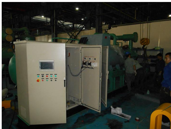
Figure 5: Generator and Synchronizing Equipment
