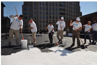
Figure 1 Volunteers painting an urban rooftop with a cool roof coating in the NYC °Cool Roofs Program (cool roof rating council)
