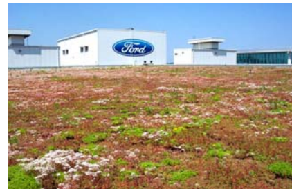
Figure 2 Ford Motor Company's River Rouge Plant Green Roof (the greenroof & greenwall projects databse)
