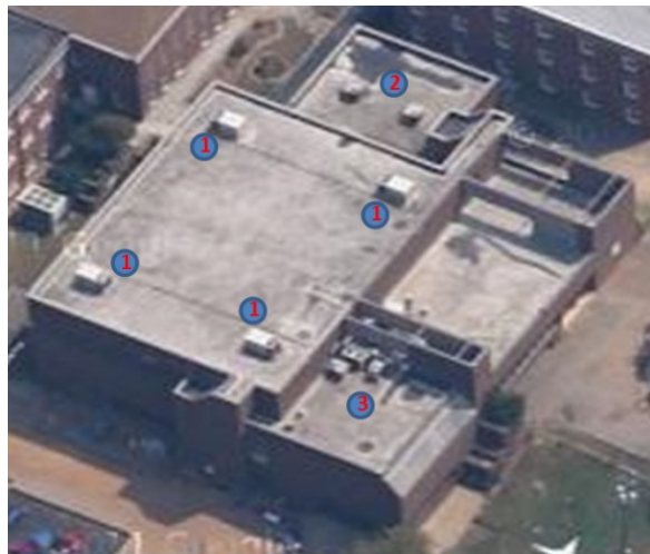
Figure 2: FLC roof view.
