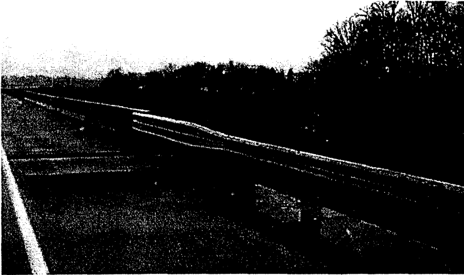
Figure 3.7: Example of Type TGB Transition
