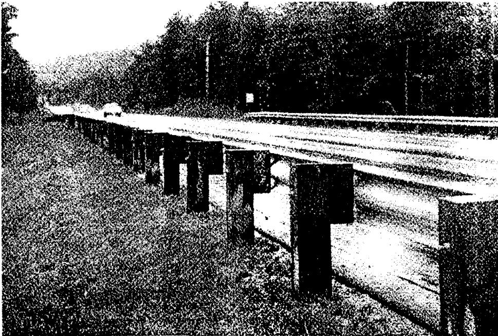
Figure 2.1: Example of Blocked Out W-Beam Approach Rail
