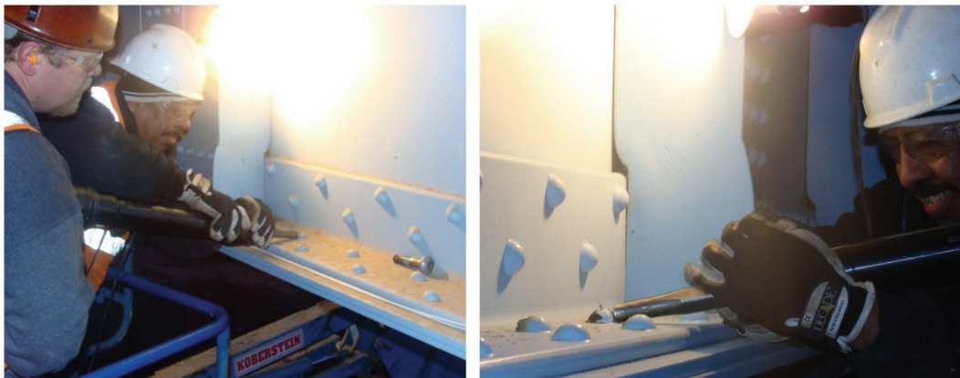
Figure 3.38 Rivet head removal using rivet buster (courtesy of Purdue University).
