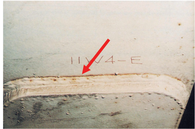
Figure 3.33 Cover plate with weld at termination.
