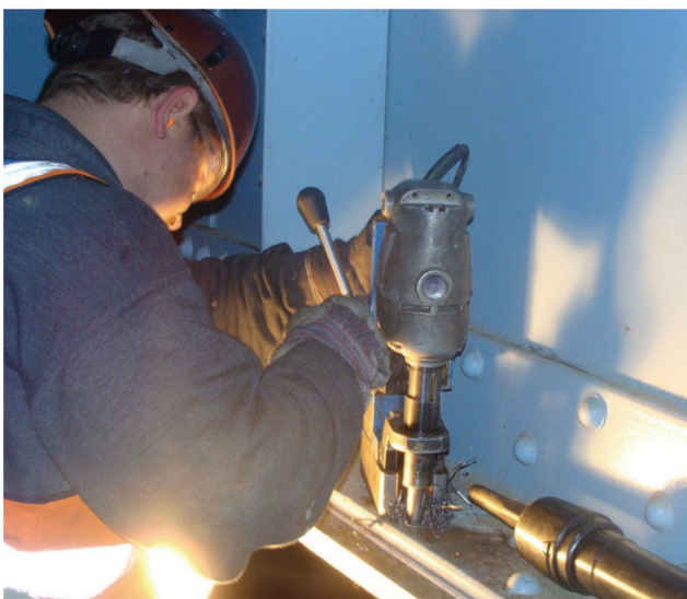
Figure 3.40 Drilling out center of rivet (courtesy of Purdue University).
