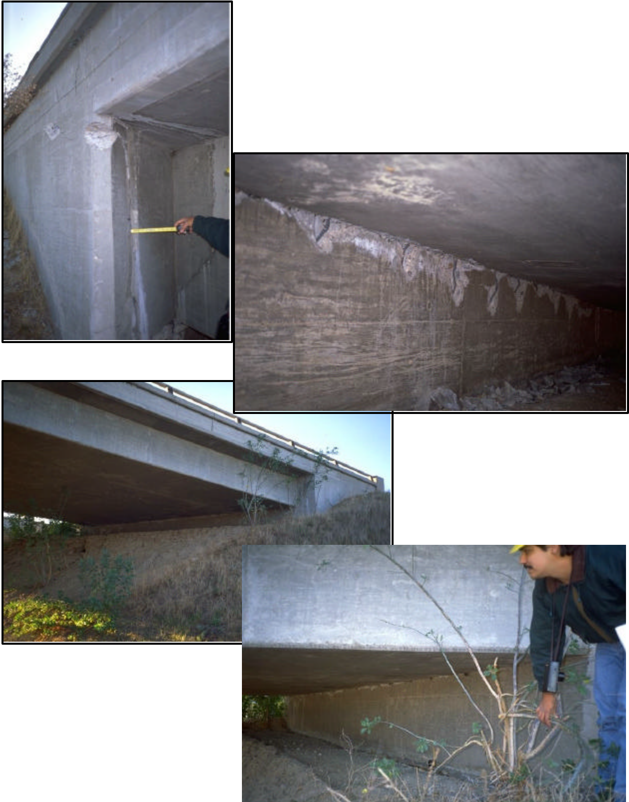
FIGURE 8.23 Different views of the superstructure of the bridge (11)
