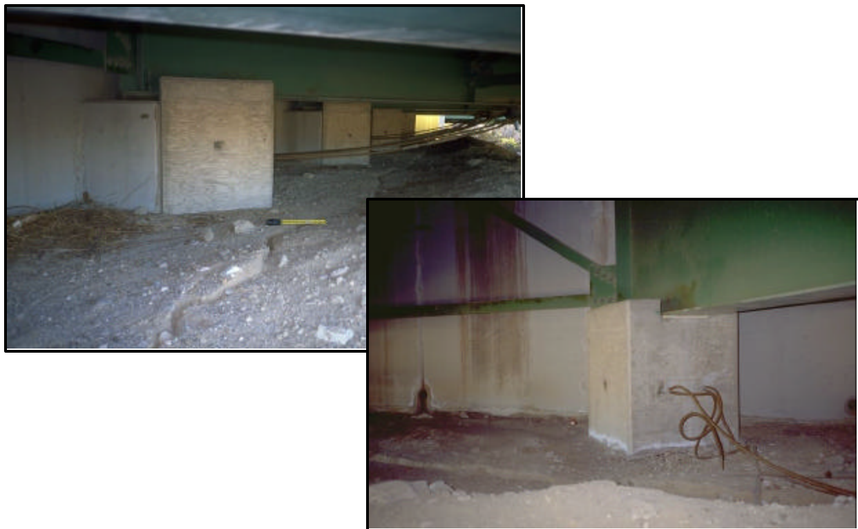
FIGURE 8.9 View of substructure and soil of the bridge (11)
