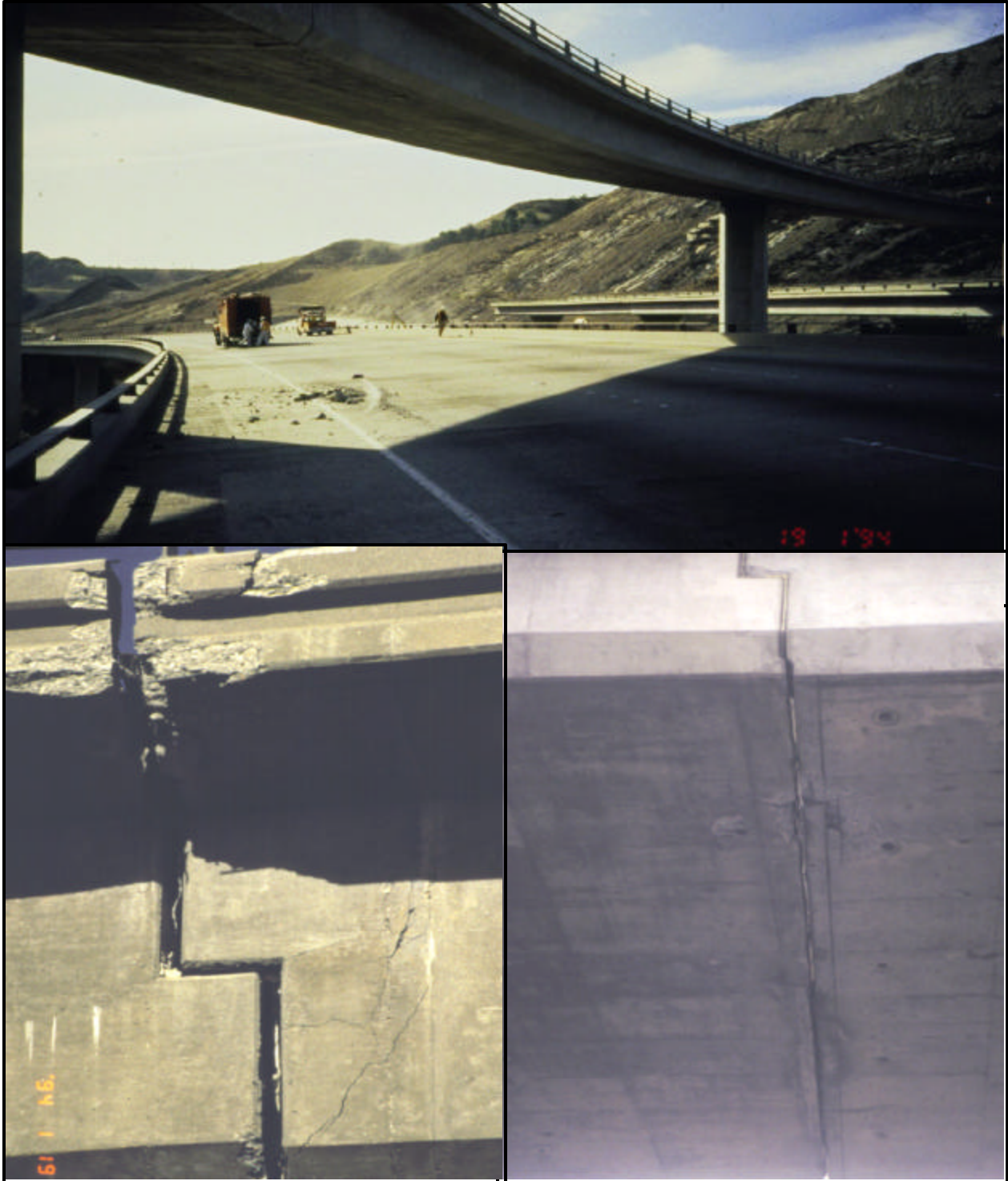
FIGURE 8.17 Different views from the superstructure of the bridge (11)
