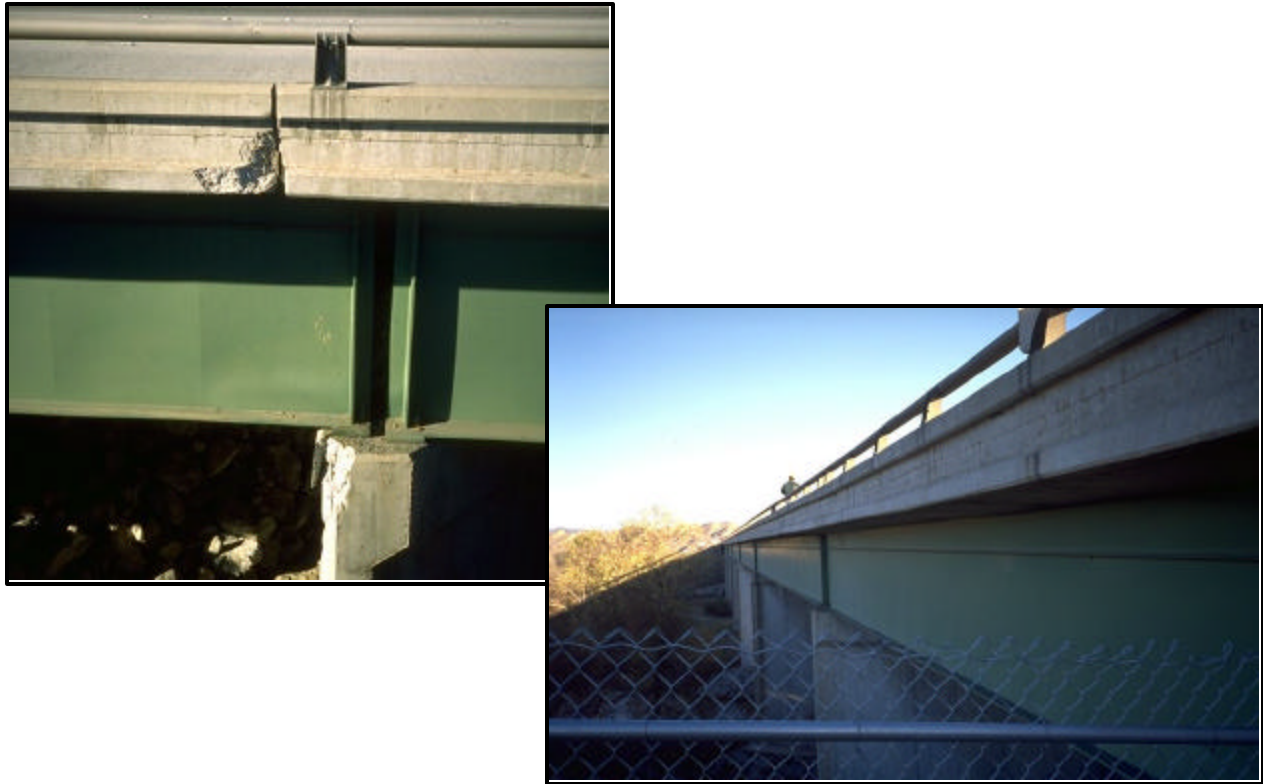
FIGURE 8.3 Different views of bridge superstructure (11)
