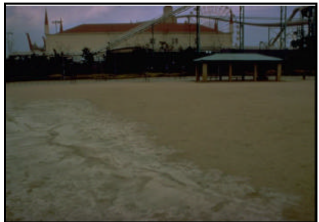
FIGURE 5.81 Sand boils and ground cracks after Kobe EQ 1995 (11)
