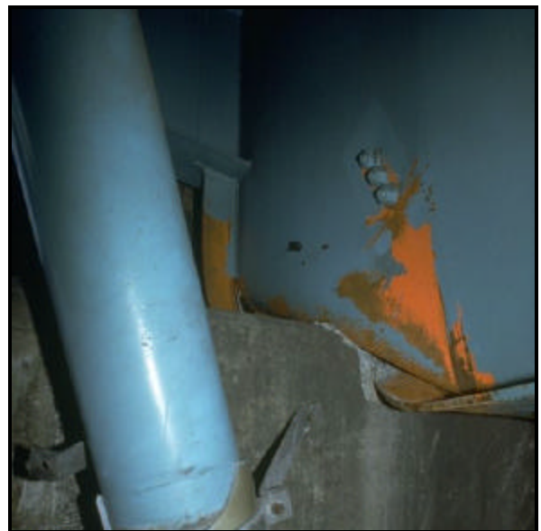
FIGURE 5.72 Pounding of steel girder to the abutment (11)
