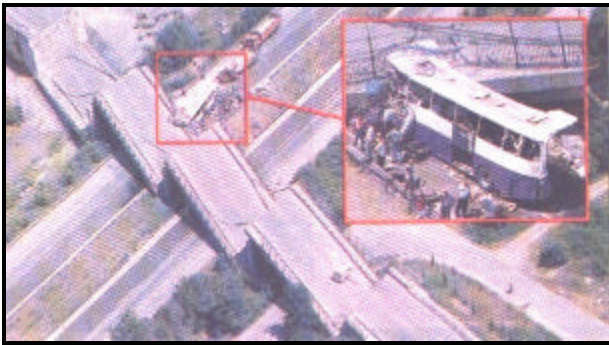
FIGURE 5.5 Failure of a prestressed concrete box beam bridge after Izmit EQ 1999 (10)
