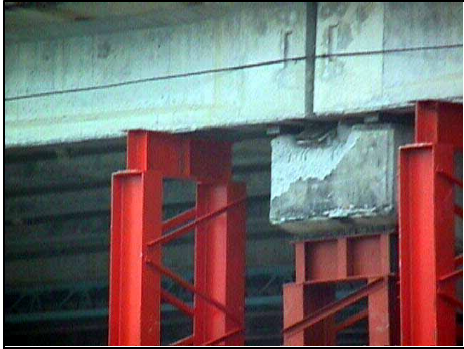
FIGURE 7.3 Temporary shoring of bridge after Taiwan Earthquake 1999 (11)
