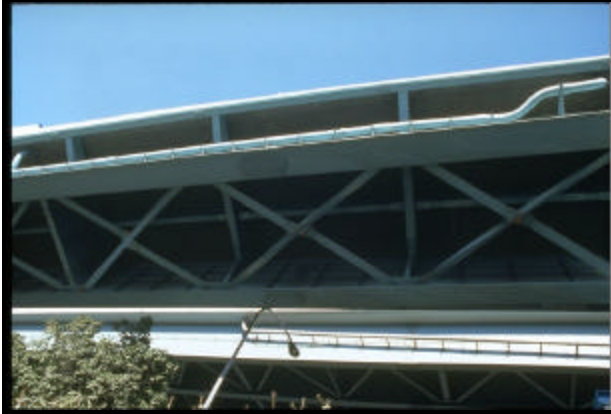
FIGURE 5.67 Twisted steel braces (11)
