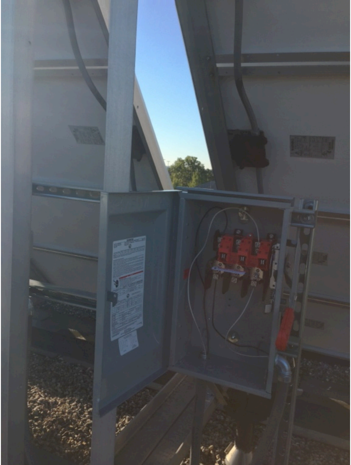
Figure C.15 Wiring Installation into DC Disconnects from Sub-Arrays
