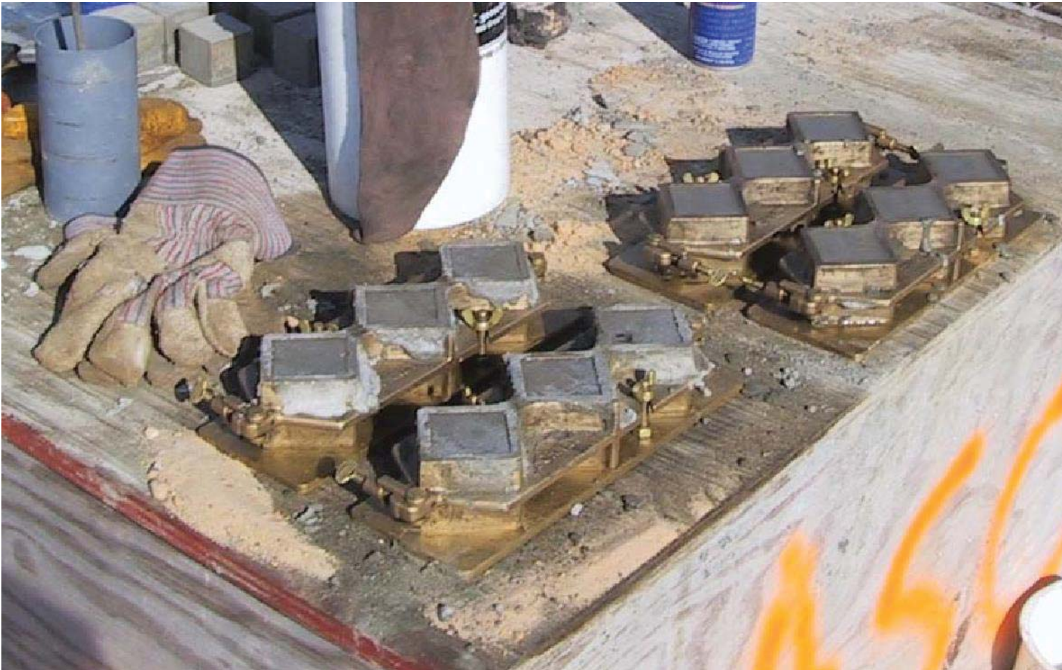
Cubes for Grout Testing
