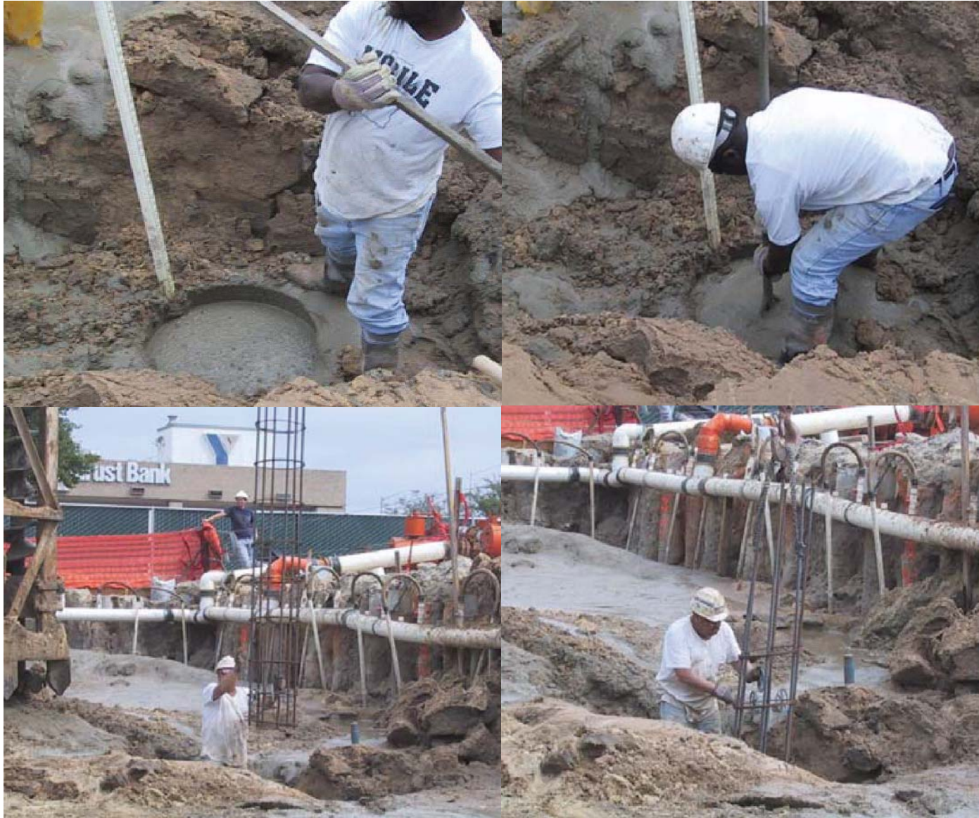
Finishing Pile and Reinforcement Placement
