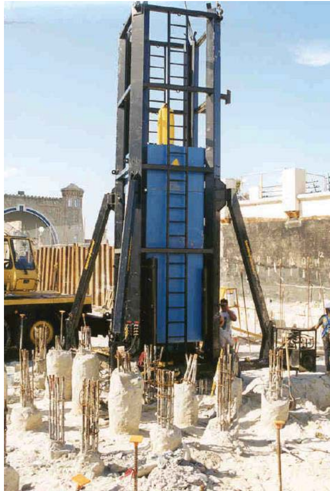
Proof Testing of Production Piles with Statnamic
