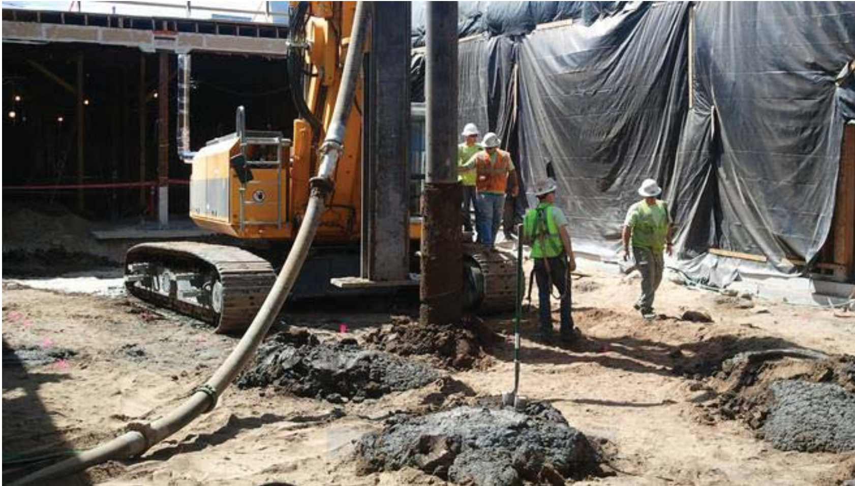
Drilled Displacement (DD) Piles
