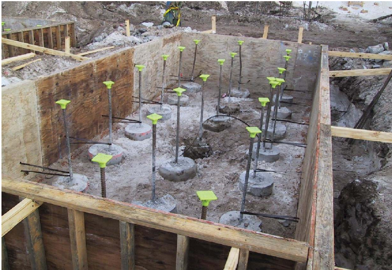
Auger Cast Piles
