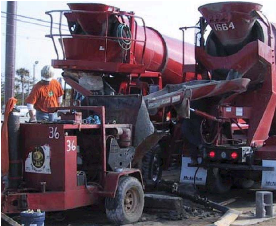
Trucks Discharging into Pump
