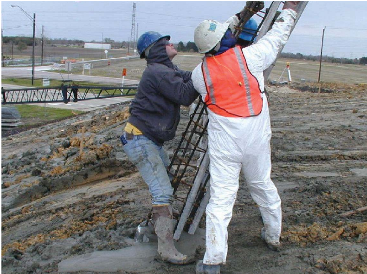
Installation of Reinforcement Cage into Battered CFA Pile
