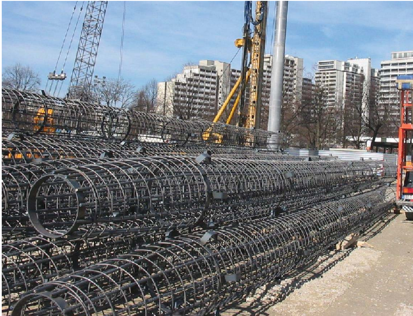
Machine-Welded Reinforcement Cage on Project Site
