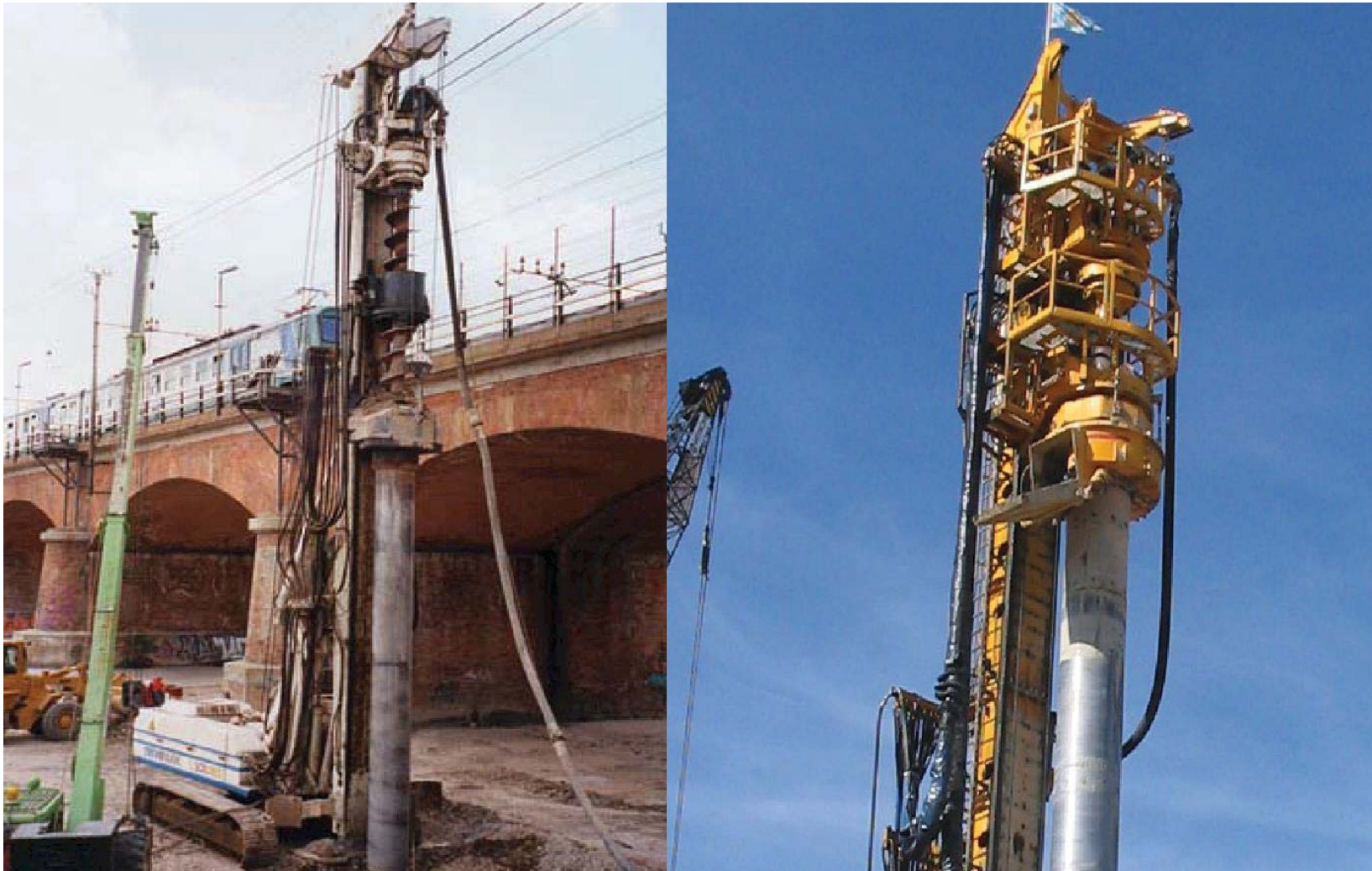
Double Rotary CFA Piles
