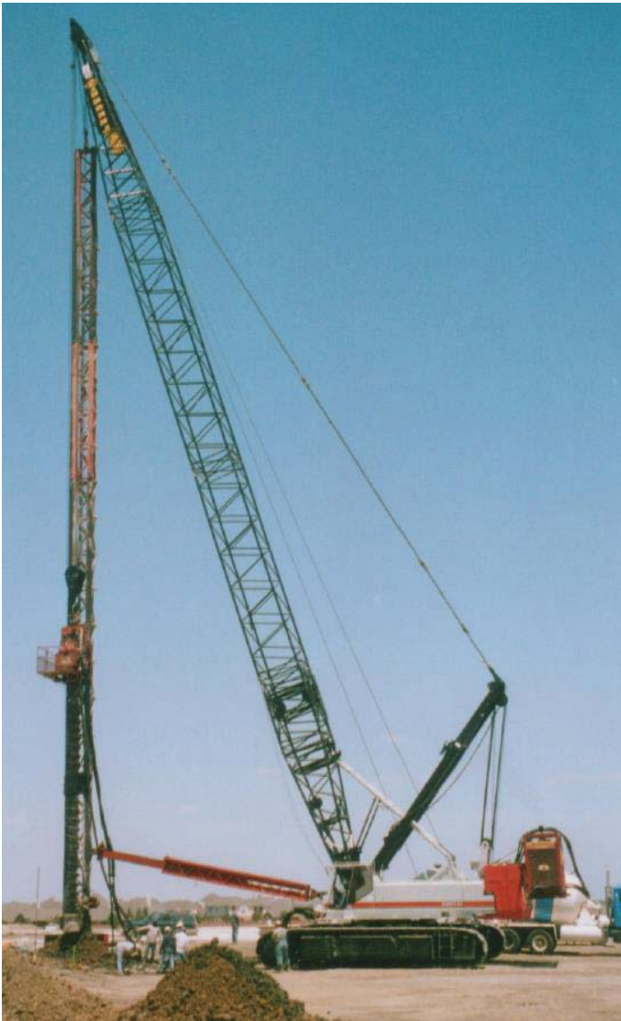
Crane-Attached CFA System
