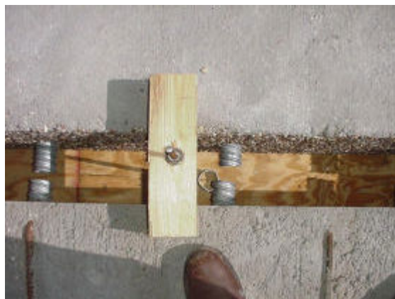
Figure 10 Wood forming of transverse panel joints.
