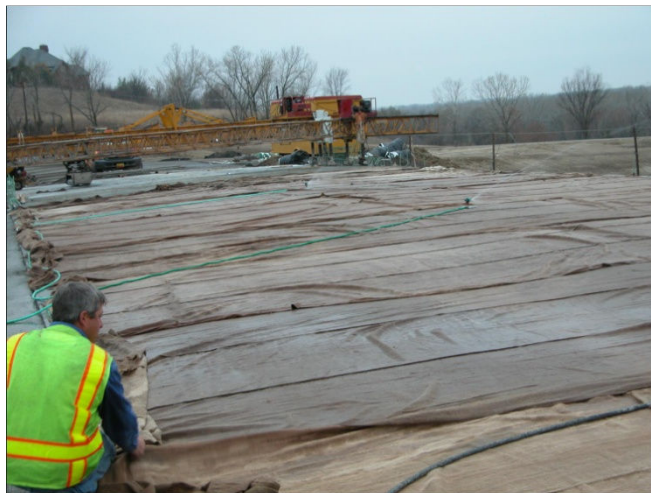
Figure 53 Curing Type K Cement Overlay.
