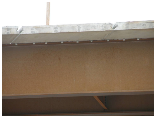
Figure 44 Panel Shear Key Configuration.
