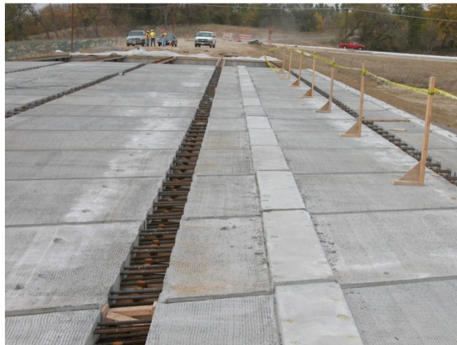
Figure 41 Another Plan View of Skyline Bridge Panels.
