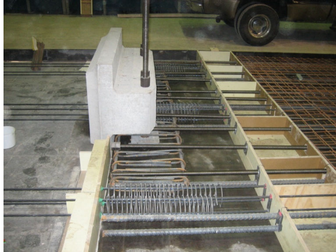
Figure 68 End of panel reinforcement.
