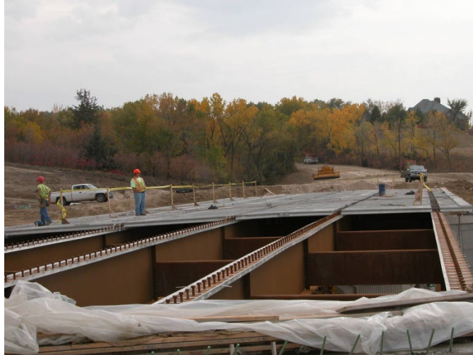
Figure 39 Plan View of Skyline Bridge after Several Panels Placed.
