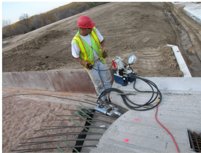
Figure 49 Post-tensioning Strands.
