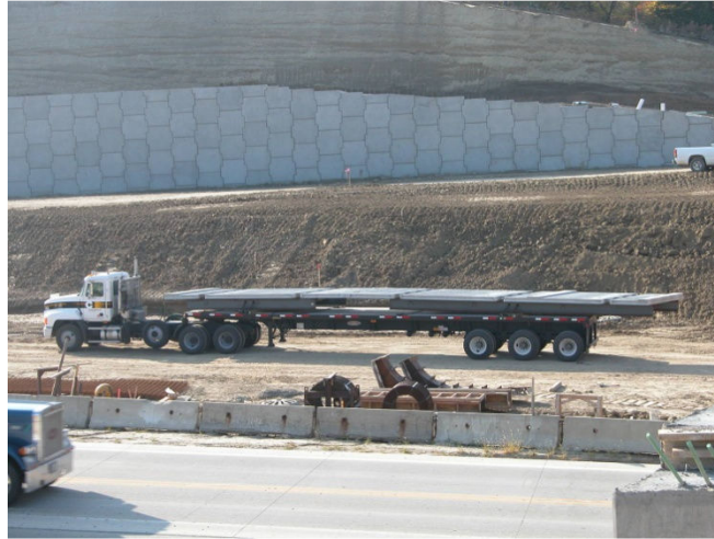
Figure 33 Skyline Bridge Panel Shipping.
