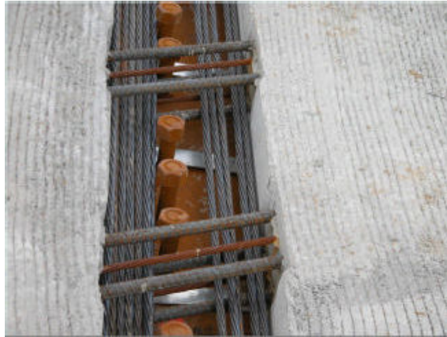
Figure 18 Strands in position in channel over girder on Skyline Bridge.
