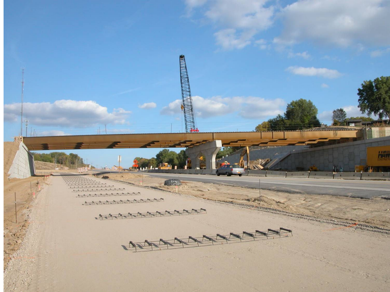
Figure 22 Skyline Bridge before Deck Erection.
