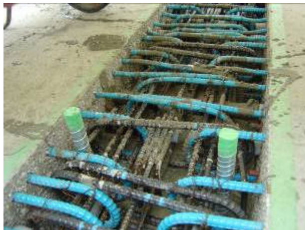
Figure 12 Longitudinal joint in Anjo Viaduct, New Tomei Expressway.
