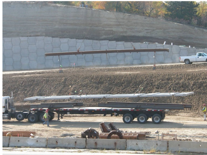
Figure 37 Erecting a Skyline Bridge Panel off the Truck.
