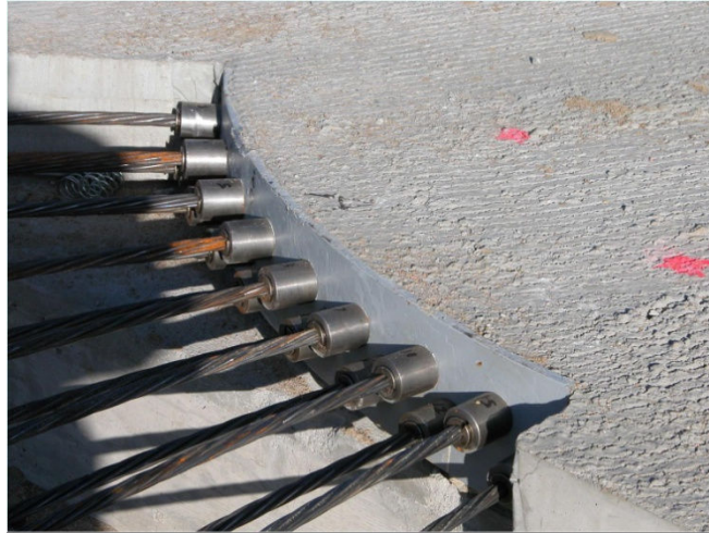
Figure 48 Strands Anchored with Chucks.
