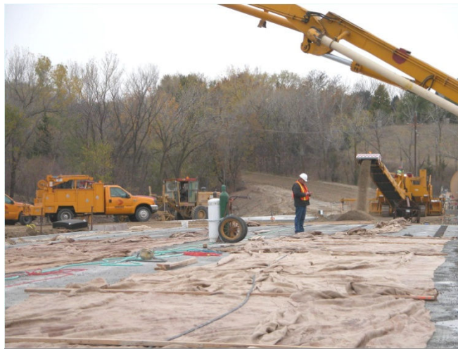
Figure 52 Curing Post-tensioning Channels.
