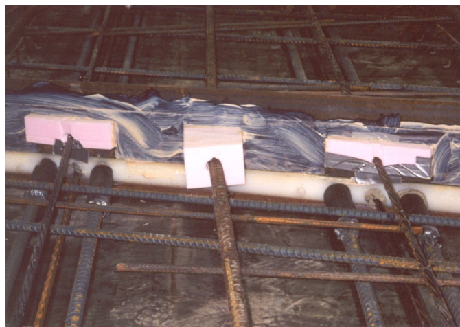
Figure 26 A Close View of Crown Forming Detail.
