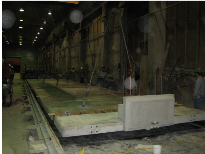
Figure 78 Lifting the precast panel from its bed.
