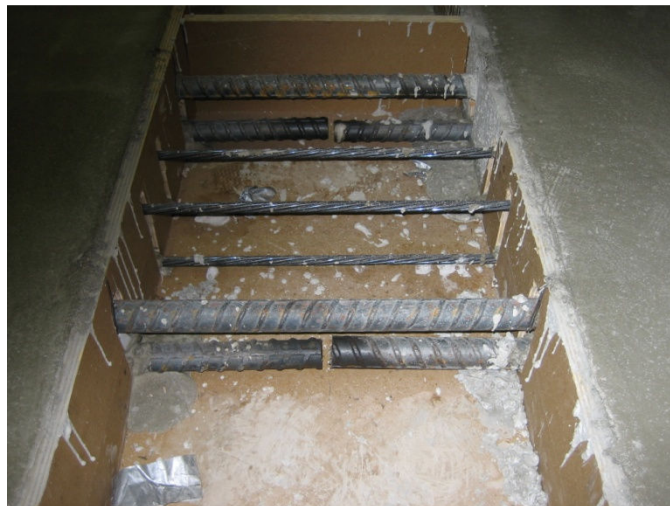
Figure 73 No. 10 bars cut at crown location.
