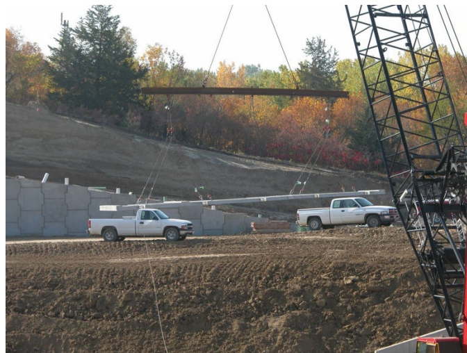
Figure 38 Erecting a Skyline Bridge Panel.
