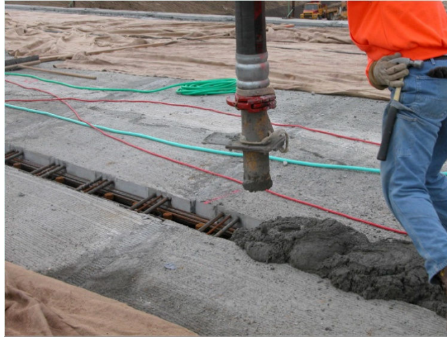
Figure 51 Pouring Post-tensioning Channel.
