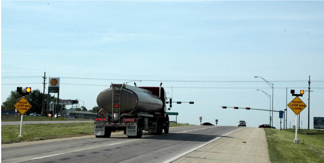
Figure 1.5 Warning Sign/Flashing Signal Heads Assembly
