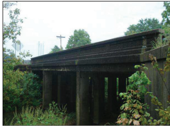
Figure 3.6 View of bridge 45-28-03529.
