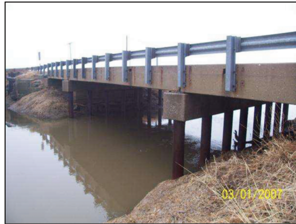
Figure 3.9 View of bridge 55-45-06258B.
