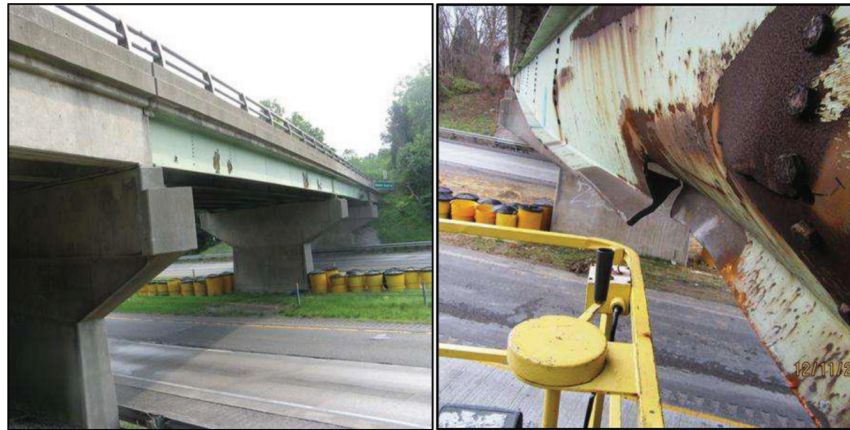
Figure 3.4 Views of bridge I65-14-0218B.
