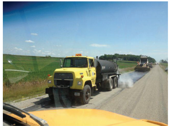
Figure 4.4 Chip seal operation (oil distributor, chipper and multi-purpose truck).
