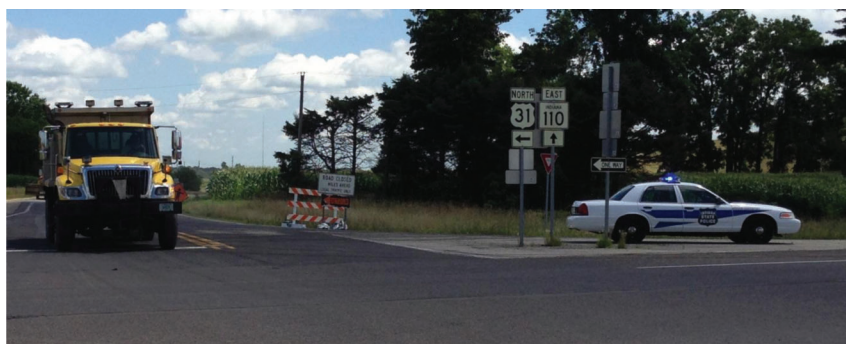
Figure 5.3 Closing a road to all but local traffic during chip seal.
