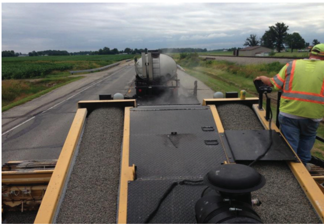
Figure 4.2 View of an oil distributor from the front of the chipper.
