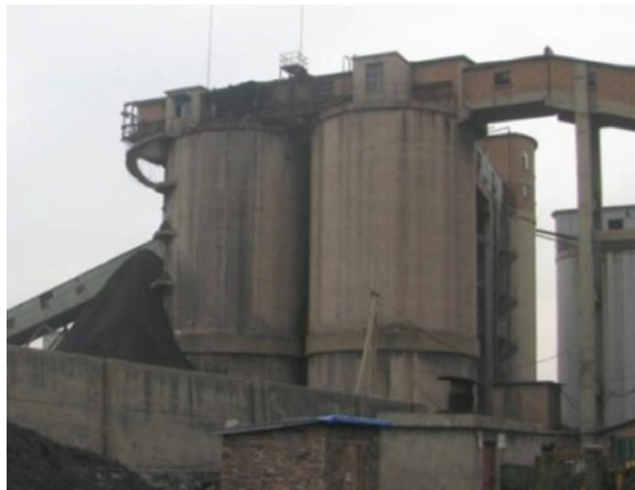
Figure 1. Panoramic view of the bunker.
