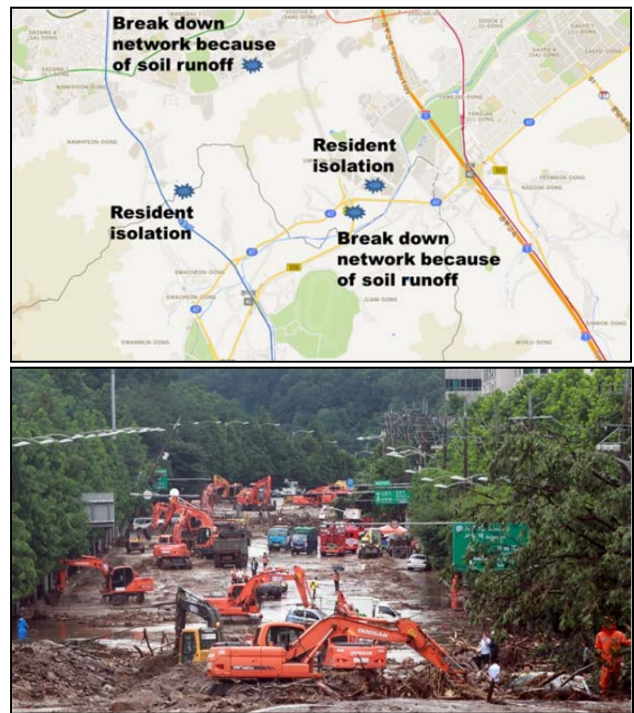
Figure 5. Mt. Umyeon landslide
