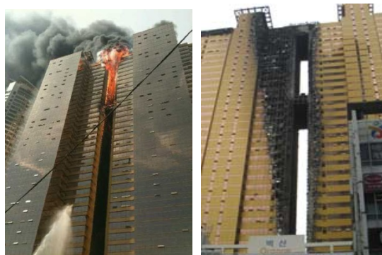
Figure 1. Fire in a high-rise building using the composite material
