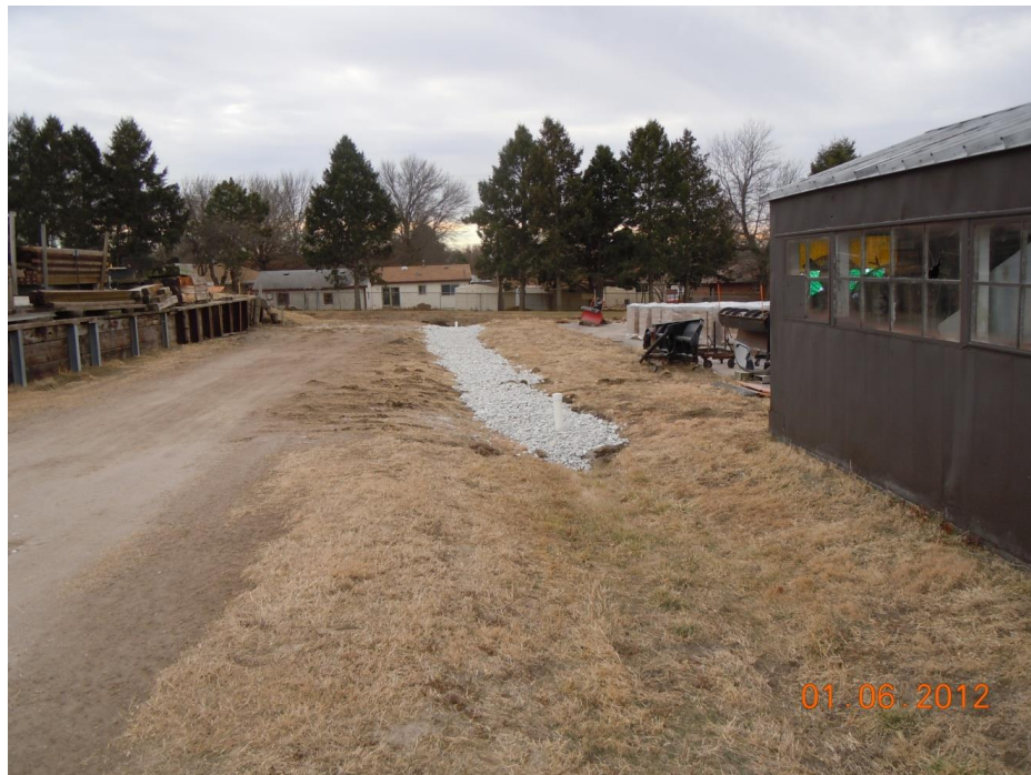
Figure B.5 Infiltration trench after construction
