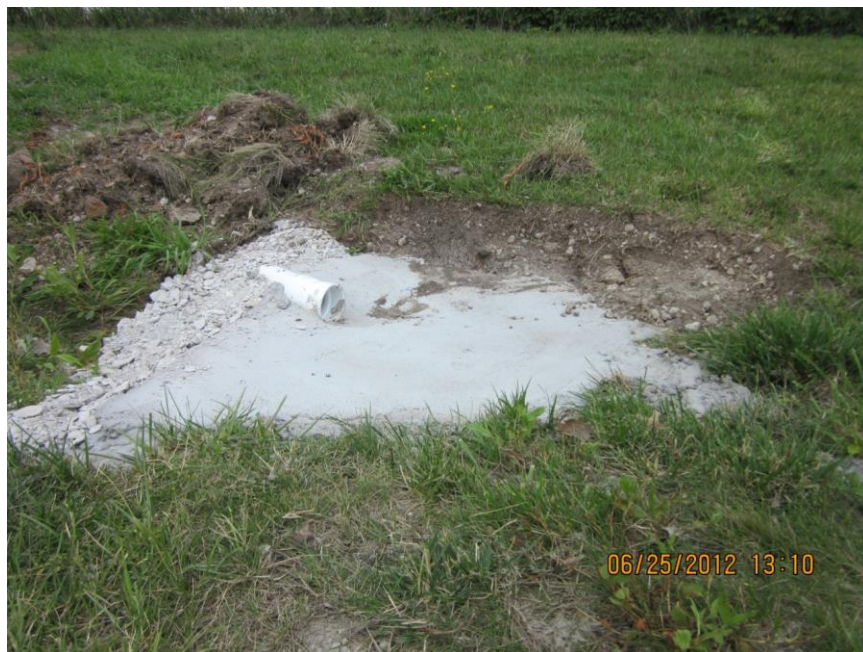
Figure B.9 Bioretention diversion after construction
