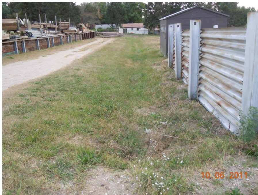
Figure B.4 Infiltration trench before construction
