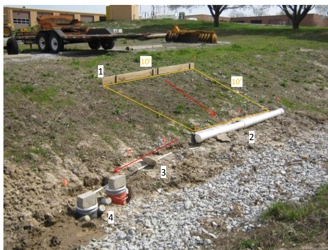
Figure 3.10 Filter trench side slope TSS collector setup
