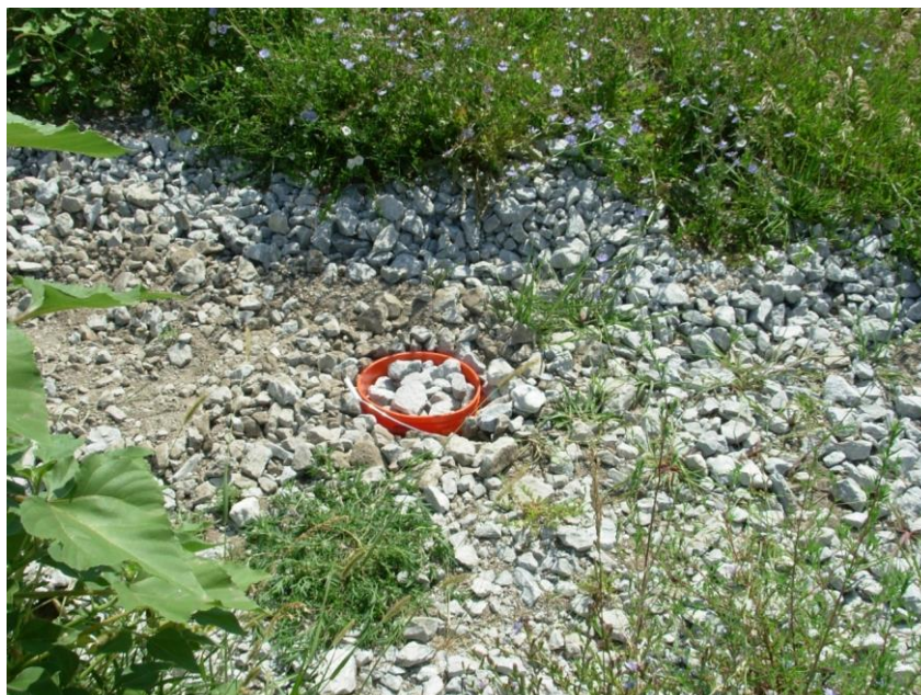
Figure B.11 Sediment bucket in infiltration trench
