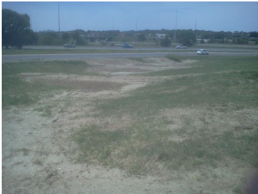
Figure B.3 Check dam filters after construction with sediment deposition
