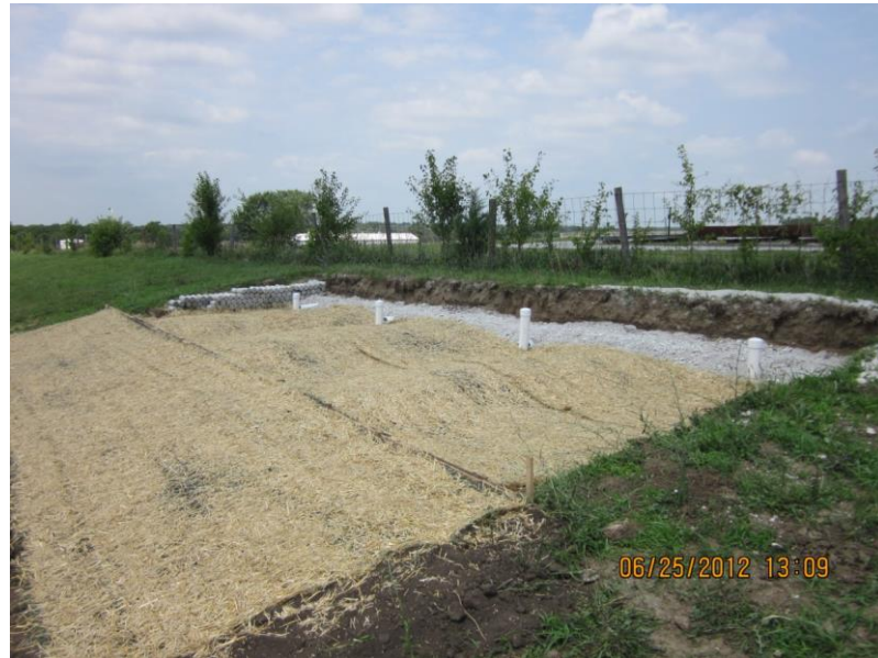
Figure B.1 Bioretention after construction
