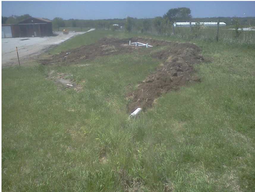
Figure B.8 Bioretention diversion during construction
