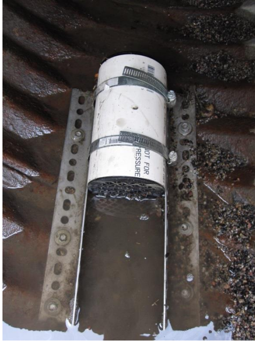
Figure 4-17 Filter trench influent sampler deployment unit
