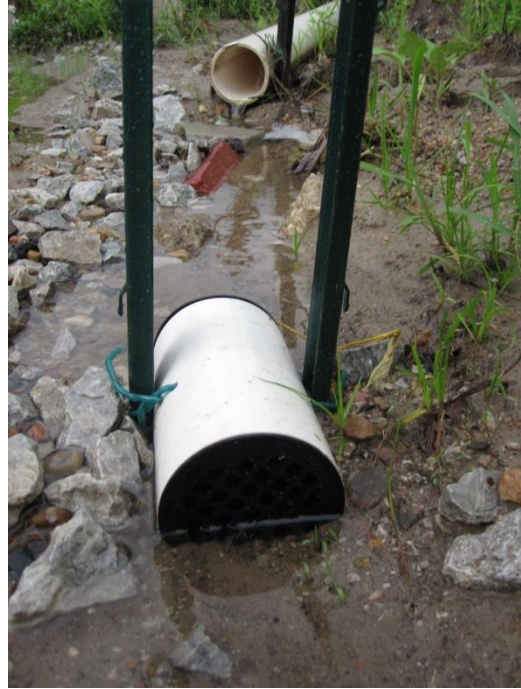
Figure 4-18 Filter trench effluent sampler deployment unit
