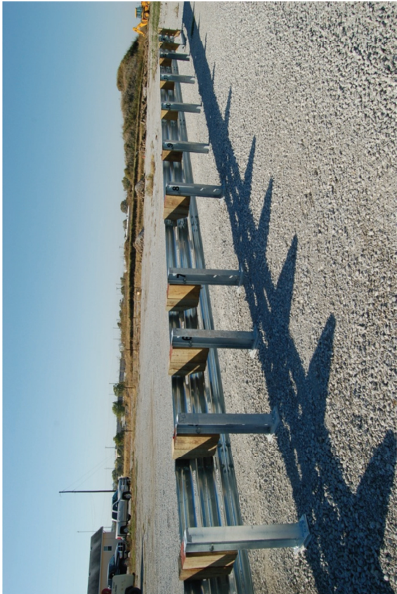
Figure 25. Test Installation Photographs, Test Nos. USBN-3 and USBN-4
