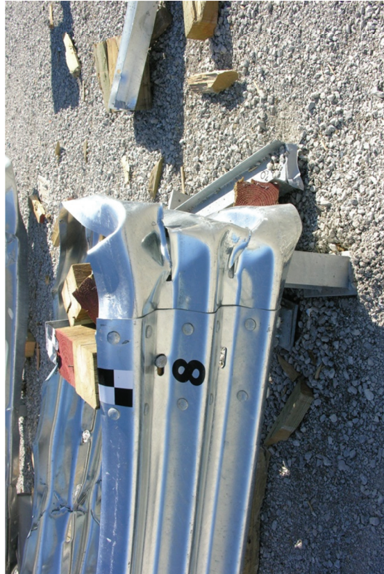
Figure 52. System Damage, Test No. USPBN-4
