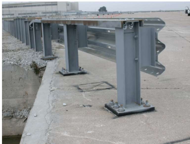
Figure 14. Anchor and Tarmac Connection Details (Design No. 1)
