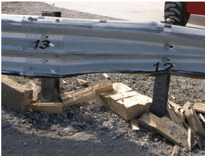
Figure 110. Post Nos. 10 through 13 Damage, Test MWT-5
