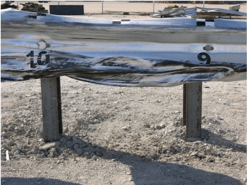
Figure 109. Post Nos. 8 through 10 Damage, Test MWT-5
