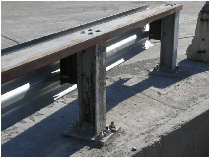
Figure 97. Anchor and Tarmac Connection (Design No. 3)
