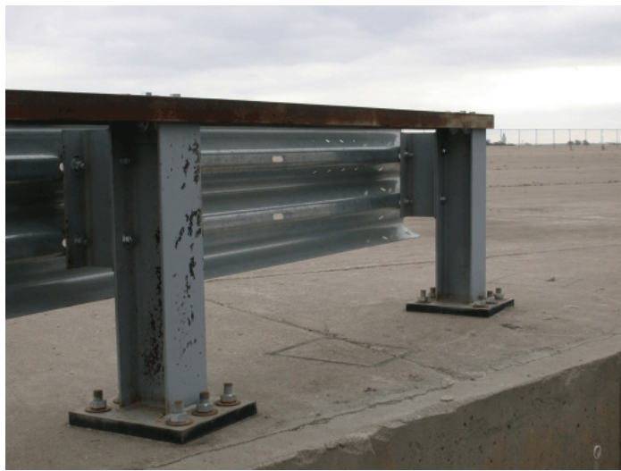
Figure 62. Anchor and Tarmac Connection (Design No. 2)
