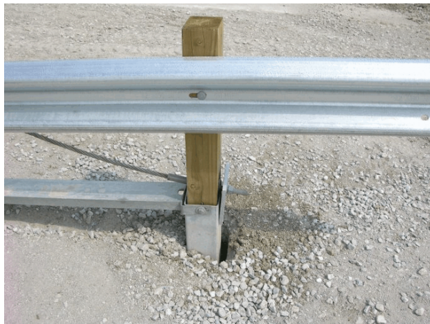
Figure 41. Downstream Anchorage Damage, Test No. MGS221-1
