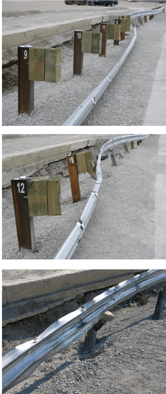
Figure 59. System Damage, Test No. MGS221-2
