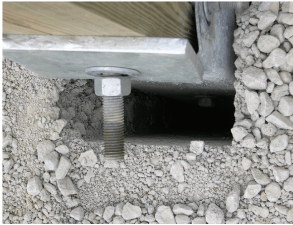
Figure 32. Anchorage Damage, Test No. MGSAS-1
