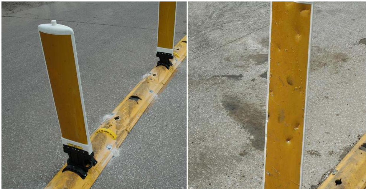
Figure 4.2. Tire tread and scuff marks on curbing installed in Fremont
