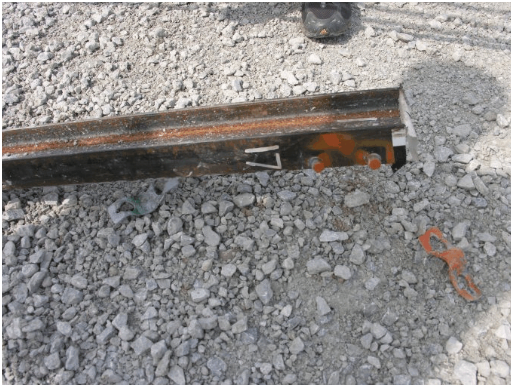
Figure 107. Post No. 17 Damage, Test No. 4CMB-3
