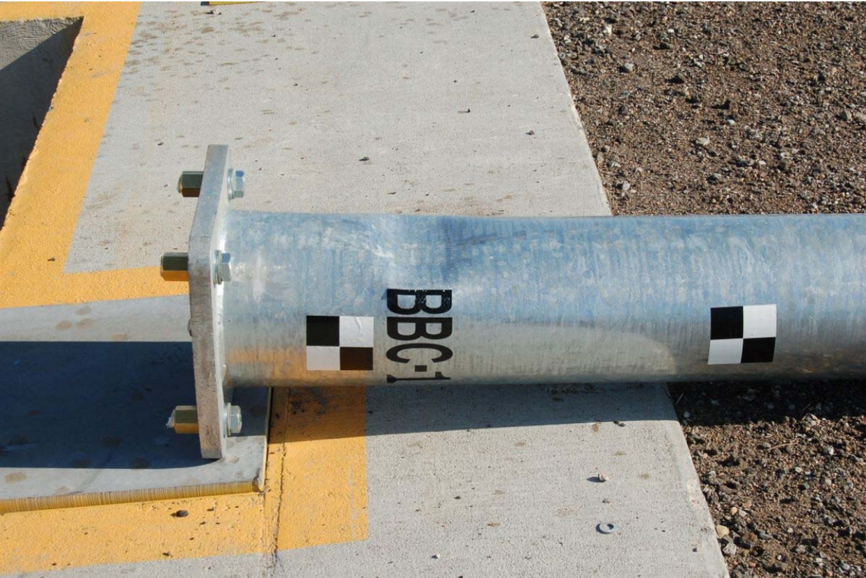
Figure 29. System Damage, Test No. BBC-1
