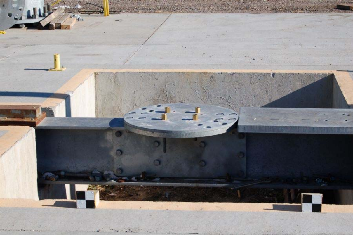
Figure 64. System Damage, Test No. BBC-6
