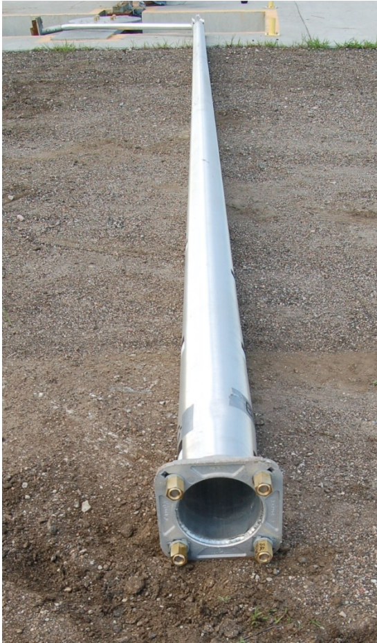
Figure 53. System Damage, Test No. BBC-5
