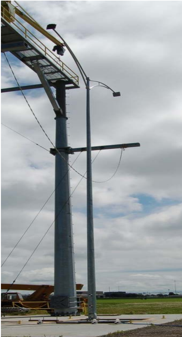
Figure 37. Assembled Test Installation, Test No. BBC-3
