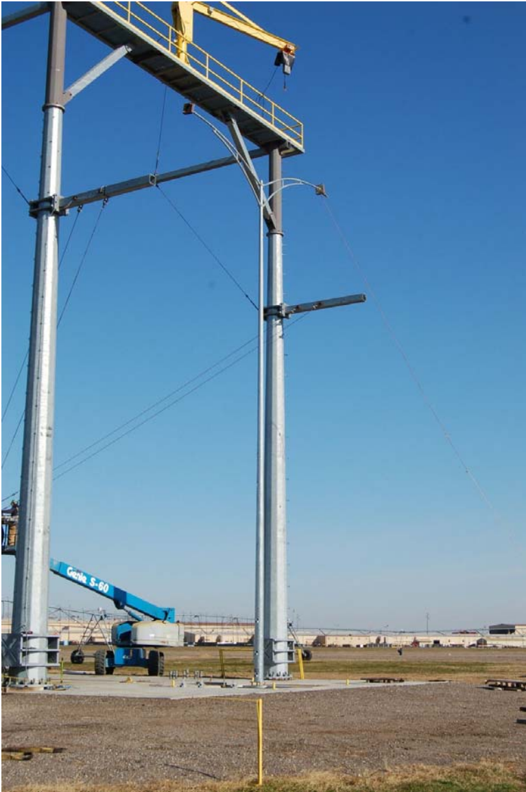
Figure 23. Assembled Test Installation, Test No. BBC-1
