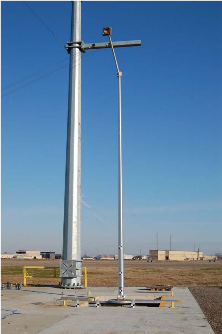
Figure 24. Assembled Test Installation, Test No. BBC-2
