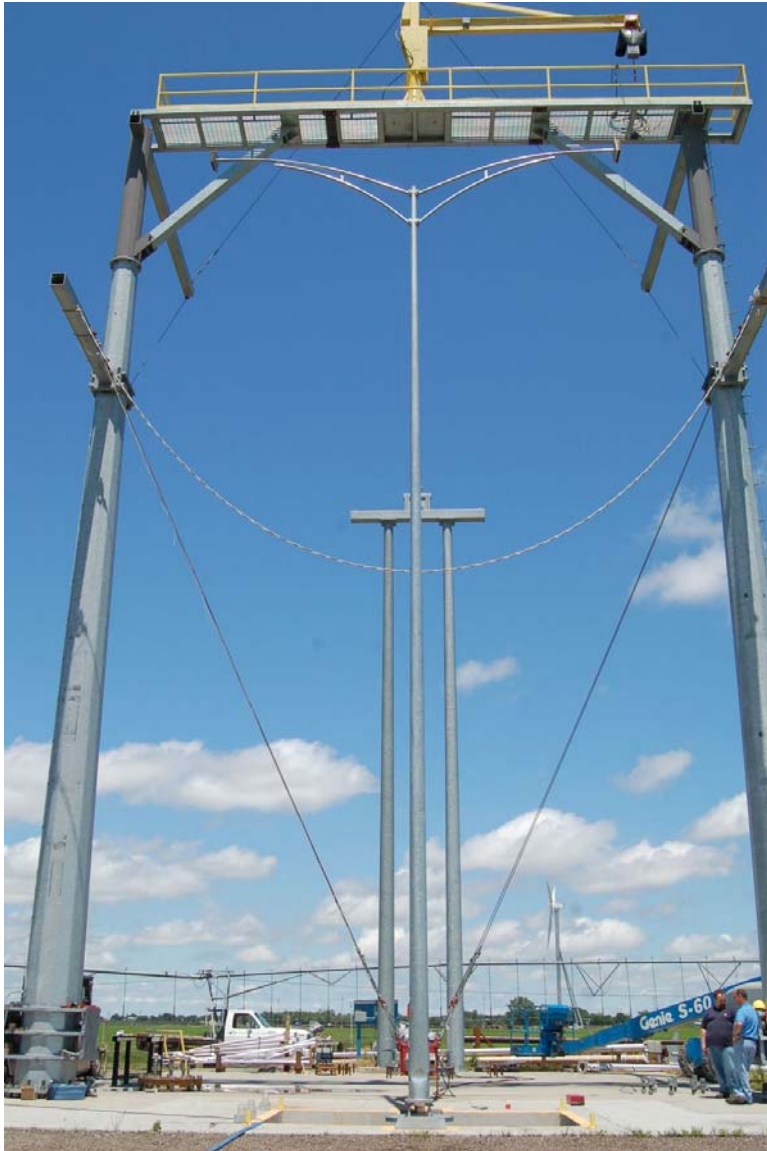
Figure 38. Assembled Test Installation, Test No. BBC-4
