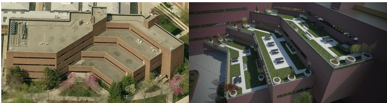
Figure 1: Knoy Hall as it currently is and what it may look like
