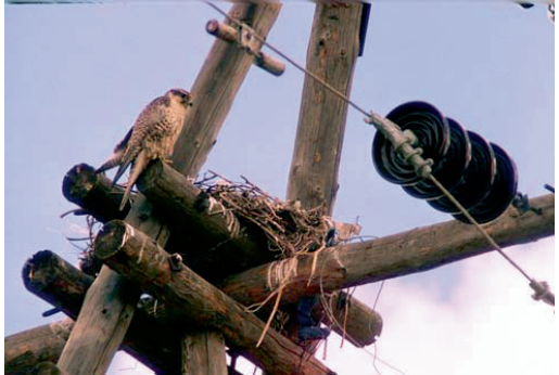
Fig. 16: Saker eyrie on wooden powerpole. In areas without cliffs, such structures probably support most nests.
