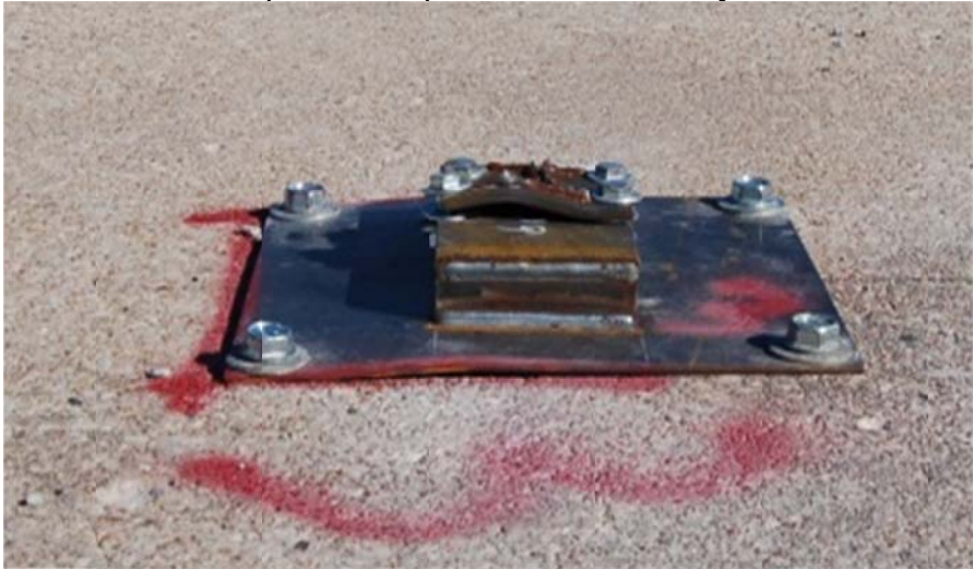
Upstream Slip Base Post Assembly
