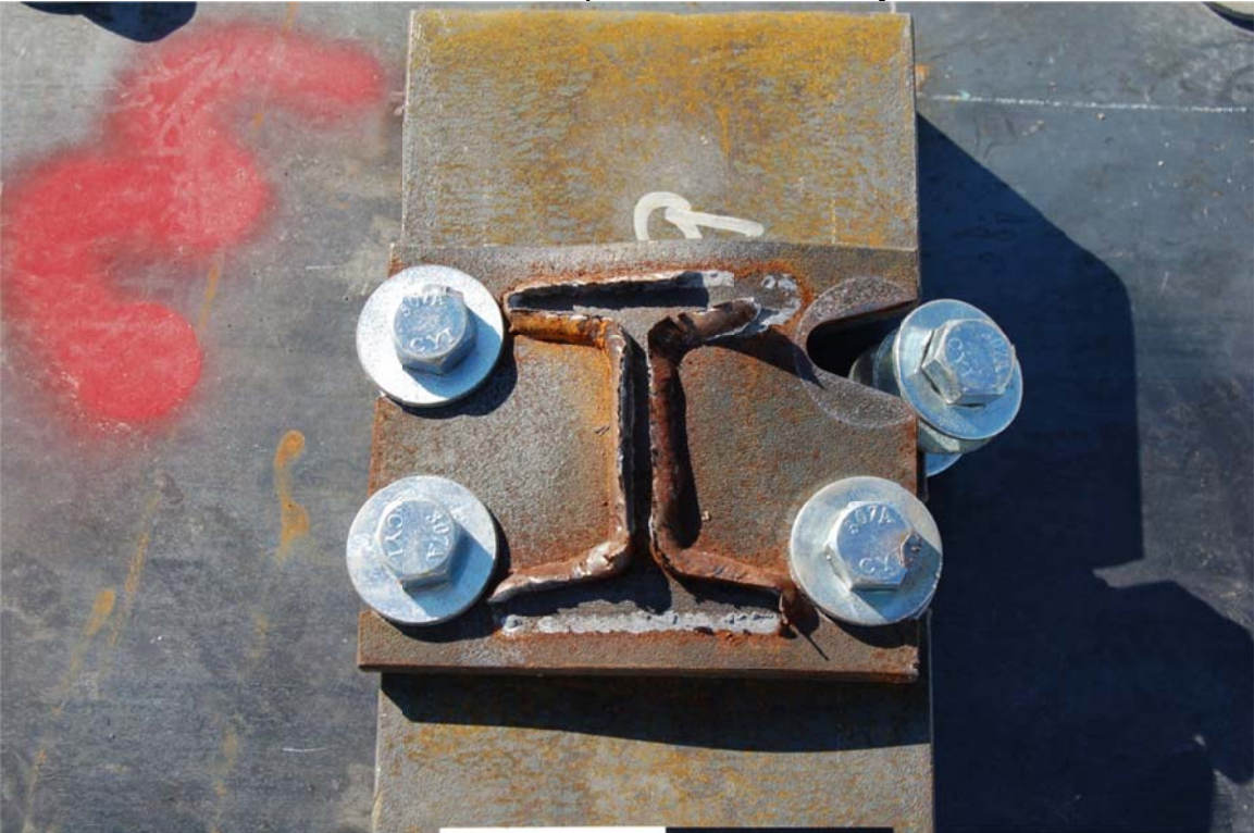
Downstream Slip Base Post Assembly
