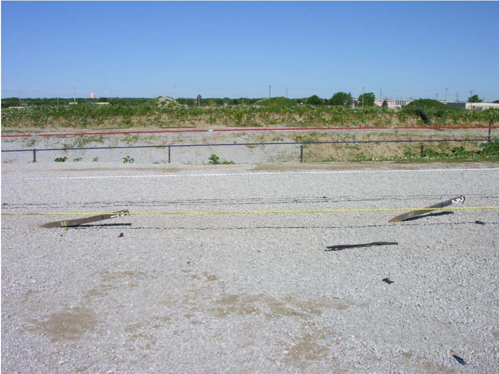
Figure 38. Post Nos. 19 through 22 System Damage, Test No. 4CMBLT-1
