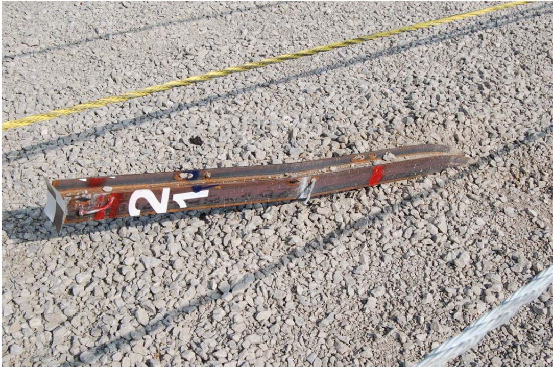
Figure 45. Post No. 21 Damage, Test No. 4CMBLT-1
