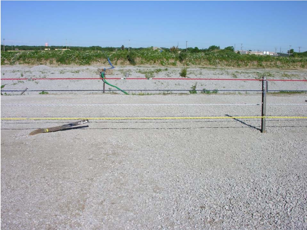
Figure 37. Post Nos. 15 through 18 System Damage, Test No. 4CMBLT-1
