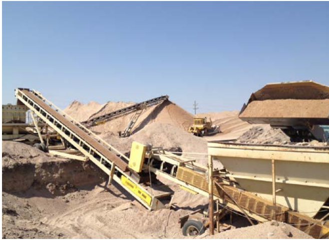
Figure 20. Aggregate Plant Site
