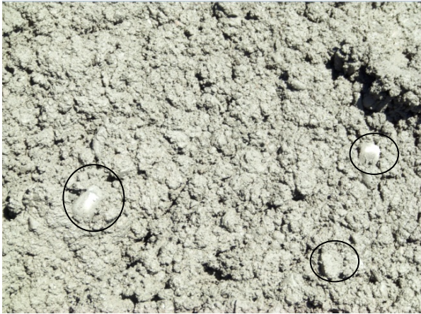
Figure 10. Aggregate's dust coating observed during paving operations.
