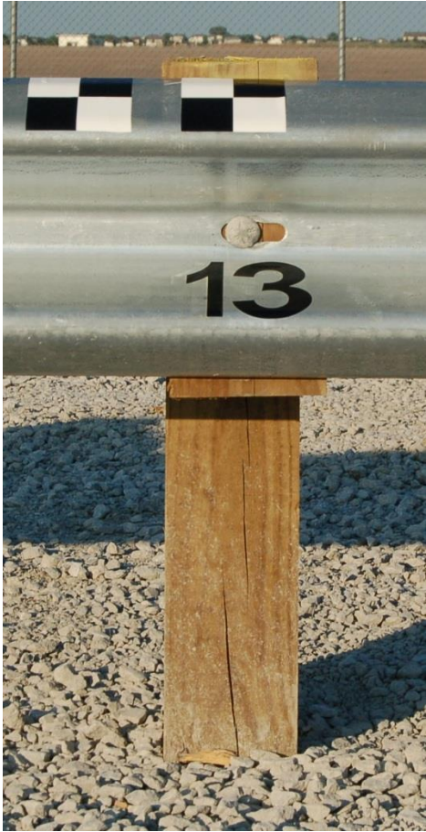
Figure 12. Test Installation Photographs, Test No. MGSSYP-1
