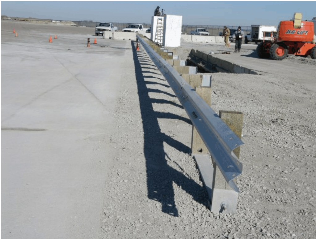
Figure 48. MGS Installed Adjacent to a 2:1 Fill Slope, Test No. MGS221-2
