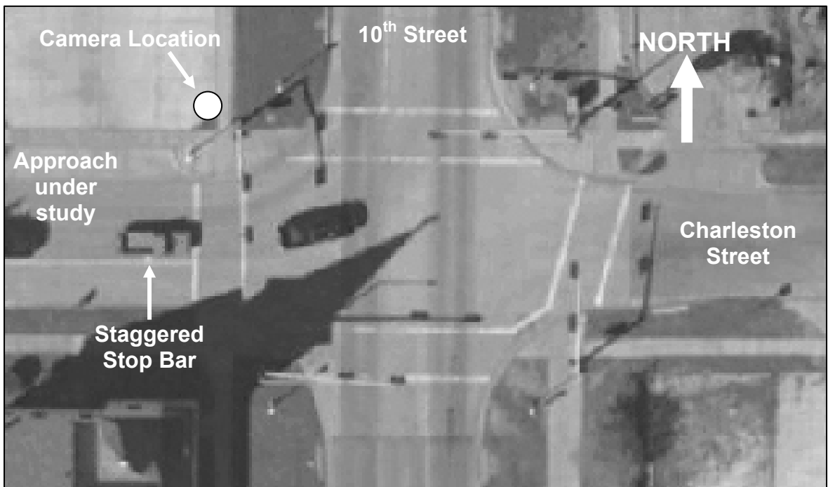
FIGURE 19 Aerial View of Staggered Stop Bar Study Site at 10 th and Charleston Sts in Lincoln, NE.
