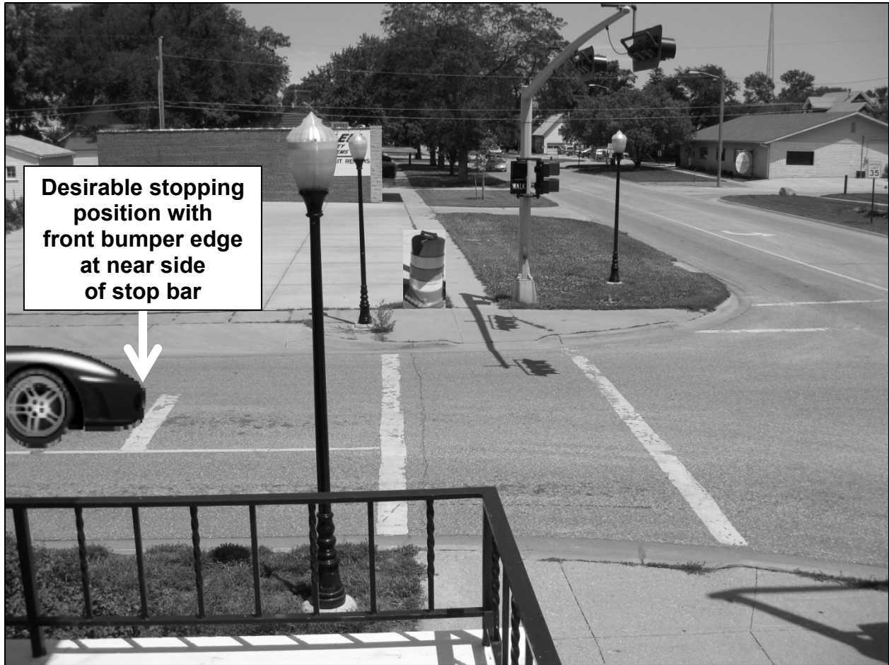
FIGURE 20 View of Staggered Stop Bar on Eastbound Approach to 10 th and Charleston Sts, Lincoln, NE.
