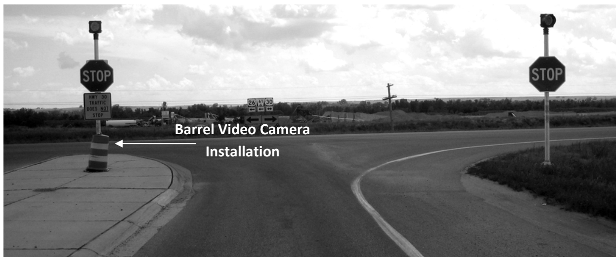
FIGURE 49 Hwy US-26 Stop-Controlled Approach to Hwy US-30
