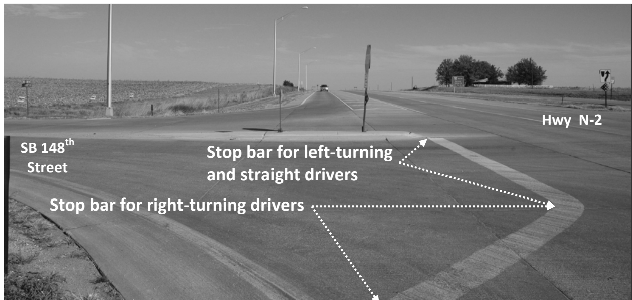
FIGURE 23 Painted Stop Bar for Both Left-Straight and Right Turning Drivers at Site 1
