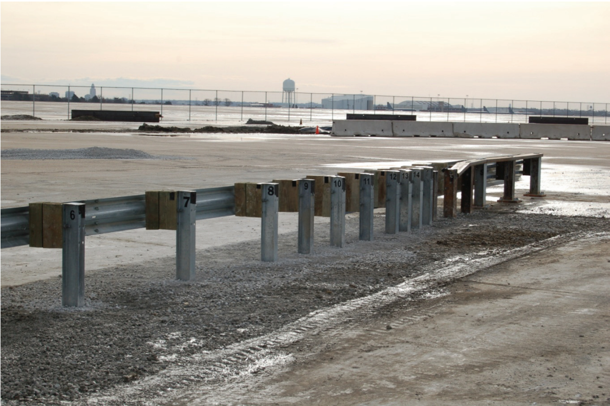
Figure 32. System Photographs, Test No. MWTSP-1
