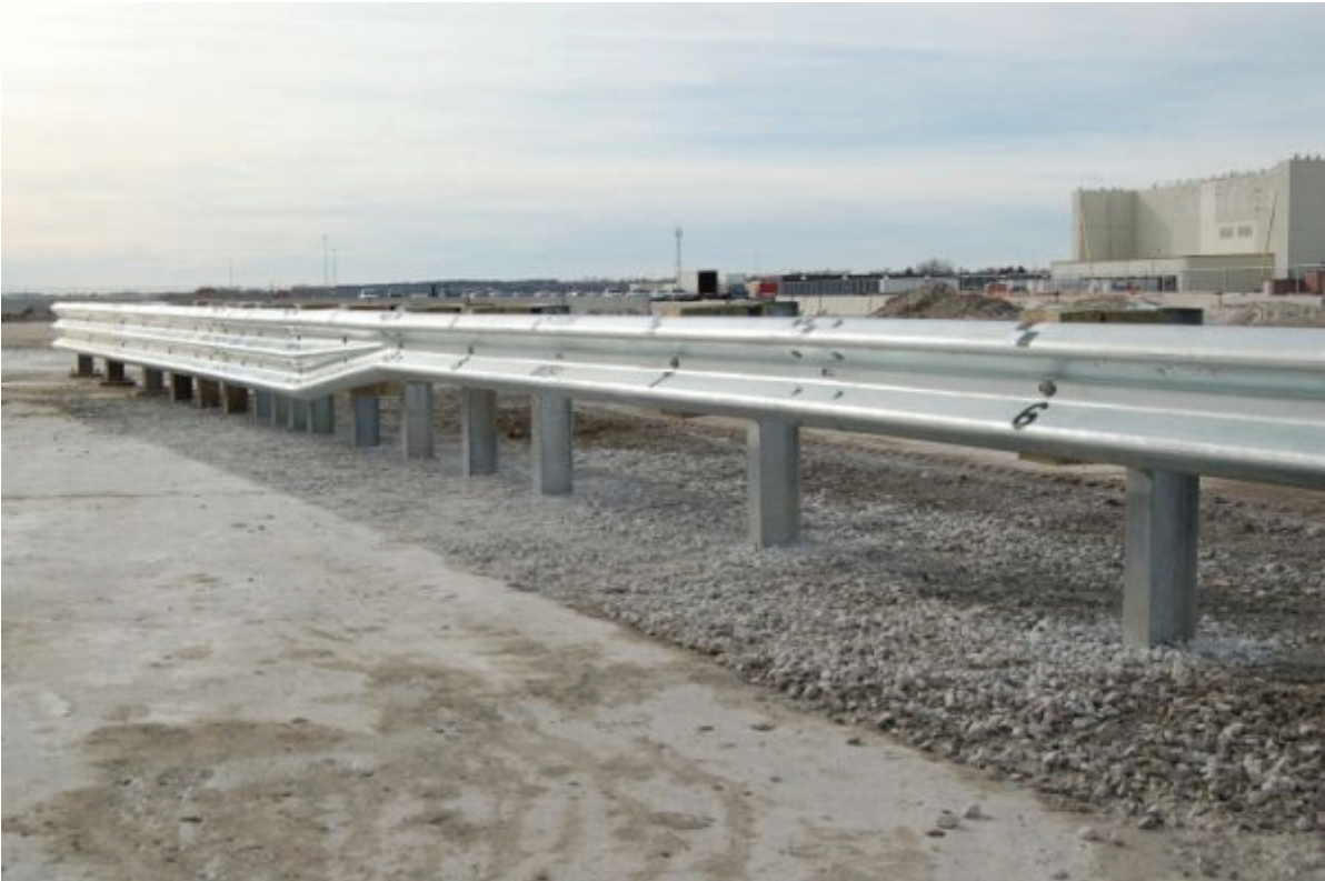
Figure 31. System Photographs, Test No. MWTSP-1
