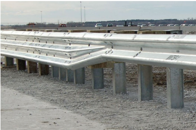
Figure 34. Transition Element Photographs, Test No. MWTSP-1
