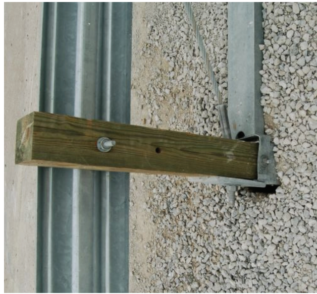
Figure 71. Upstream Anchorage Damage, Test No. MWTSF-2
