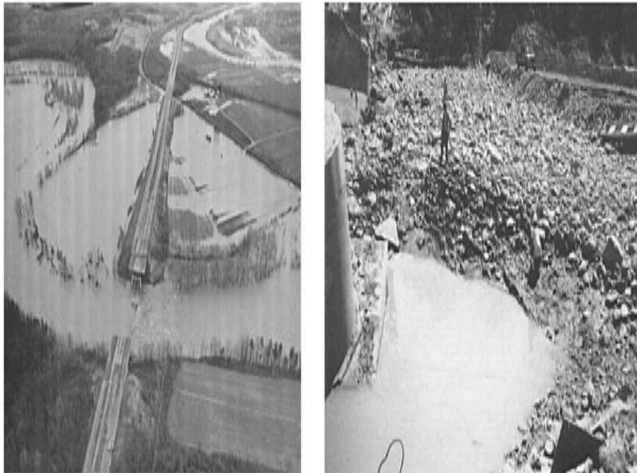
Figure 1.2 Schoharie Creek Bridge, New York, failed by bridge pier scour in glacial till in 1987 (National Transportation Safety Board, 1988)
