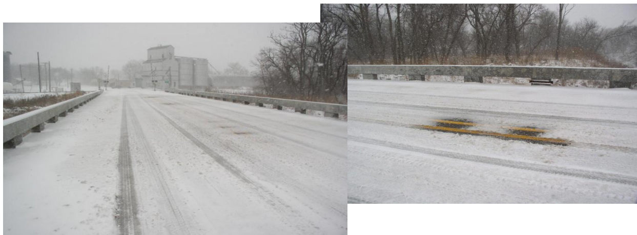
Figure 13. Hot spots along the Centerline of the Bridge Deck
