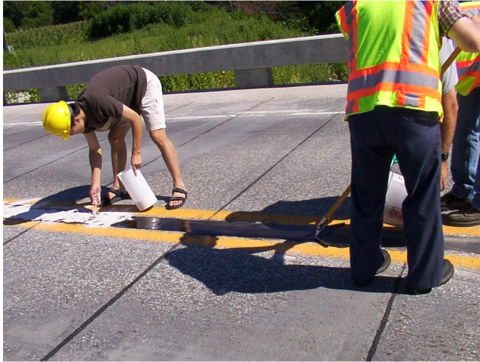
Figure 14. Application of Epoxy Coating and utility sand
