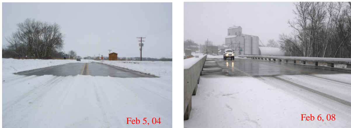
Figure 28. Roca Spur Bridge Deicing Operation
