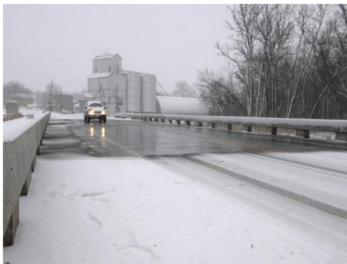
Figure 11. Ice-free Bridge Deck
