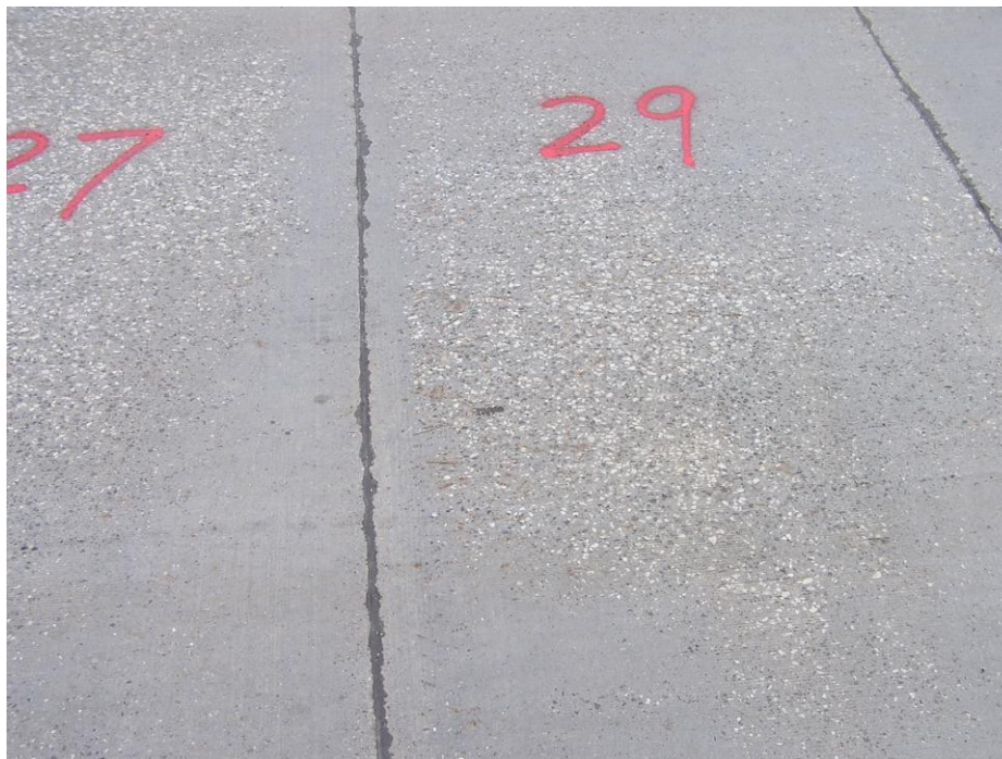
Figure 26. No Noticeable Deterioration in Westbound Lane Slabs
