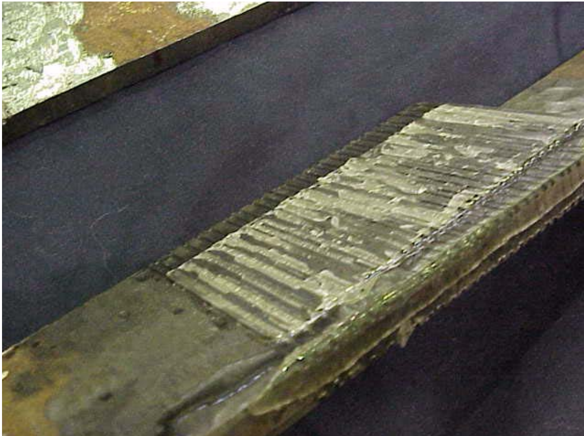
Figure 3-38: Close-up of failure
