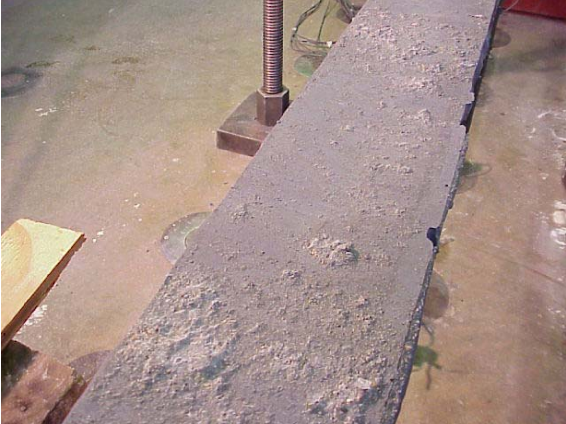
Figure 3-74: Exposed Epoxy Surface
