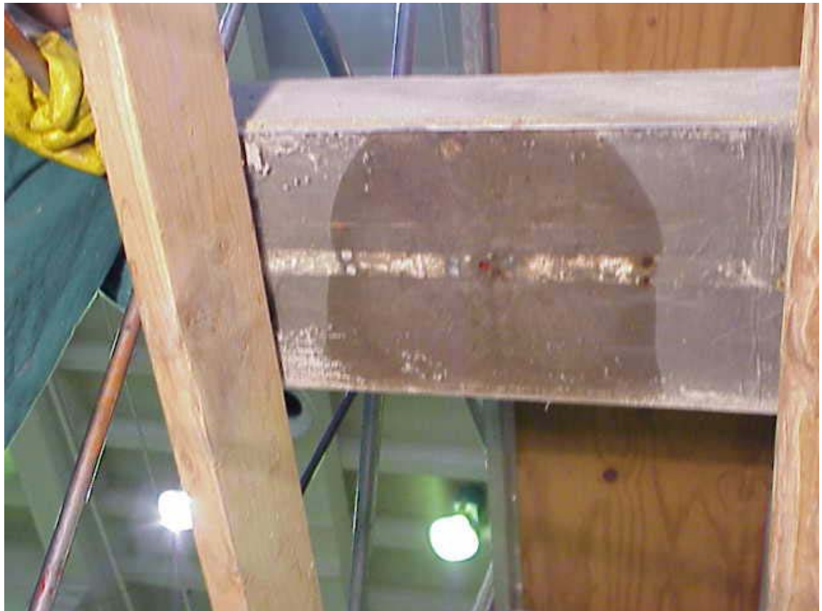
Figure 3-16: Pumping Epoxy (2)
