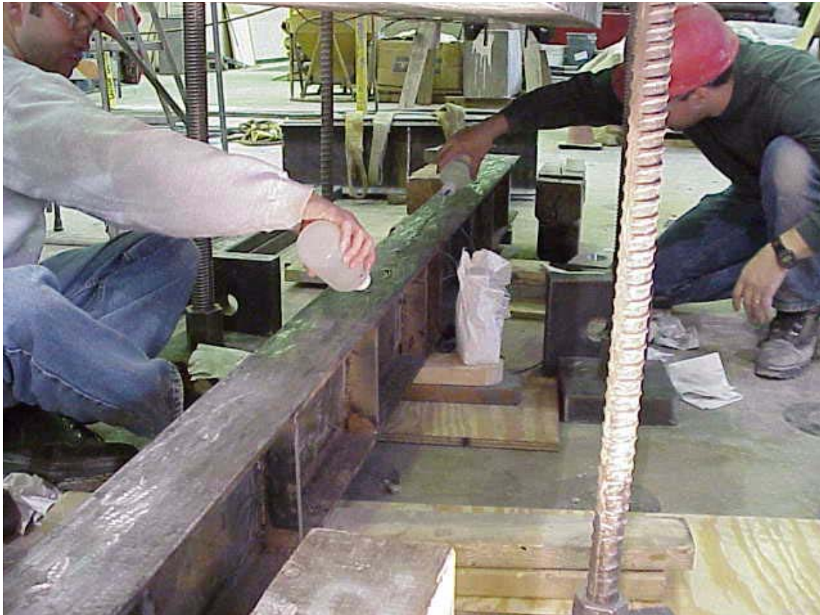
Figure 3-68: Preparation of Steel Surface
