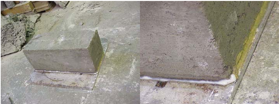
Figure 3-19: Test Setup after caulking
