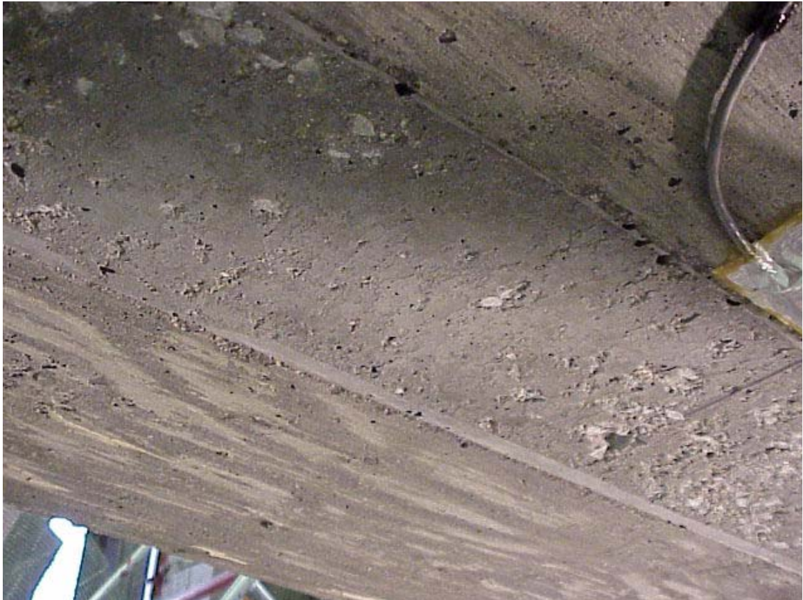
Figure 3-73: Underside of Deck after removal
