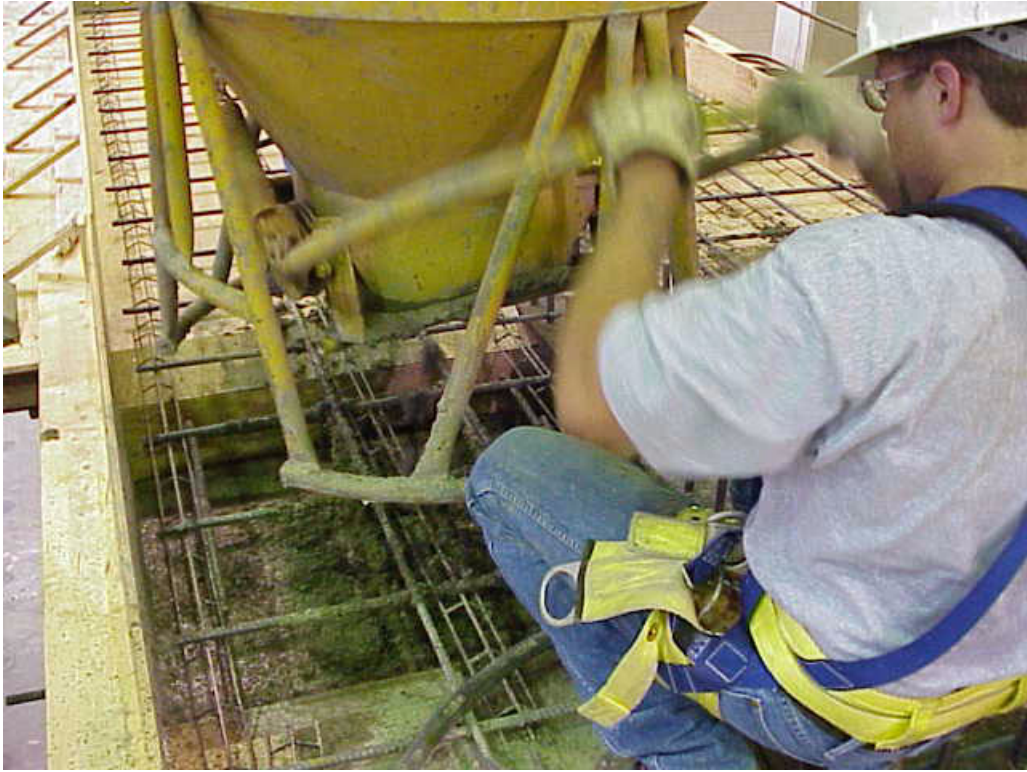
Figure 6-24: Partial Casting of the Diaphragm
