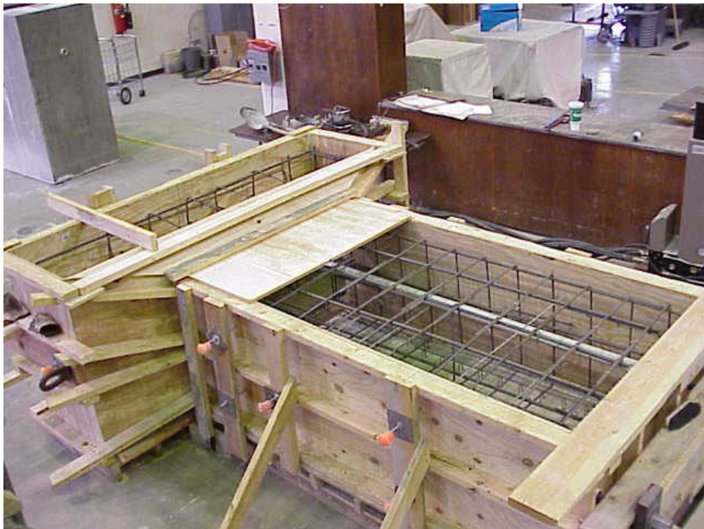
Figure 6-11: Pier Form Work Prior to Casting
