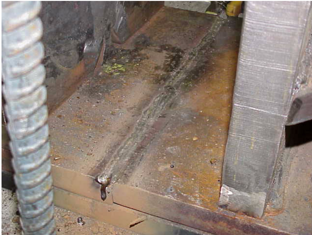
Figure 6-18: Flange Weld After Completion
