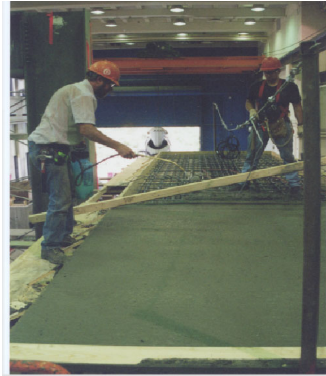
Figure 6-26: Casting of Deck Slab
