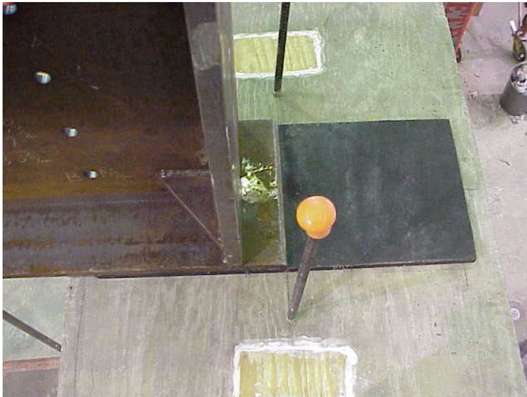
Figure 6-16: Placement of First Girder on Bearing Pad
