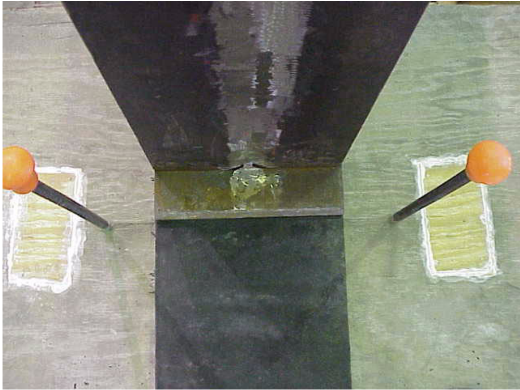
Figure 6-15: Placement of First Girder and Additional Grinding
