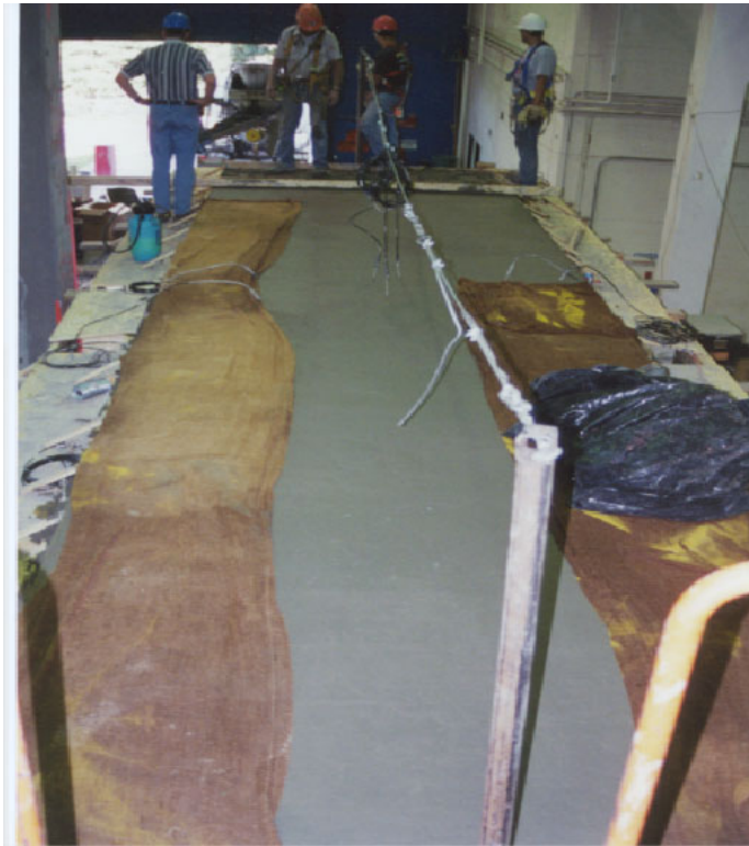
Figure 6-27: Casting of Deck Slab (Completed)
