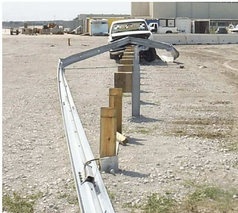
Figure 75. Vehicle Final Position and Trajectory Marks, Test NPG-3
