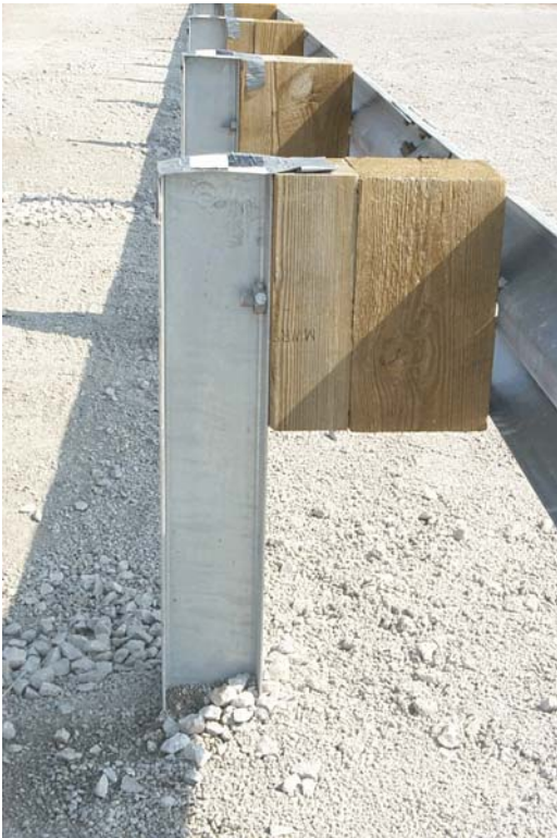
Figure 54. Midwest Guardrail System Nominal Height
