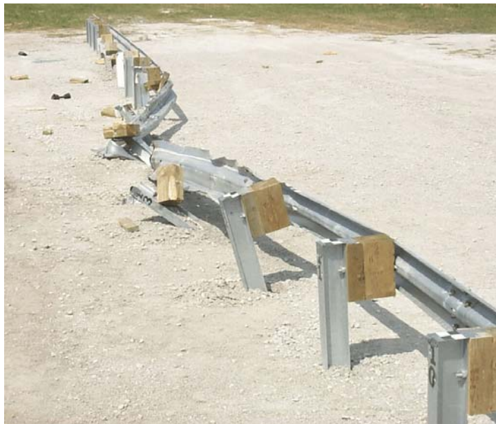
Figure 65. System Damage, Test NPG-2
