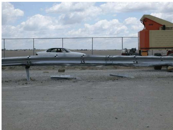
Figure 95. System Damage, Test NPG-4
