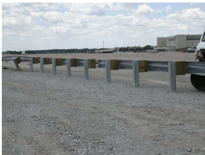
Figure 96. System Damage, Test NPG-4
