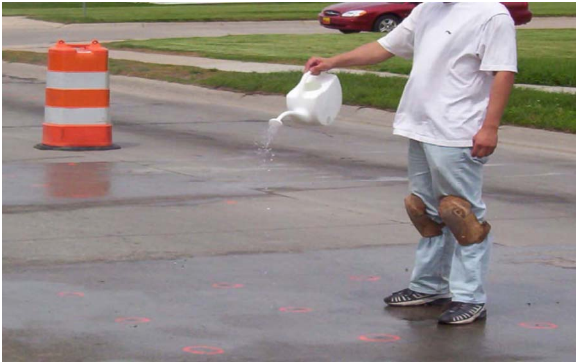
Photo No. 9 – Application of Water
