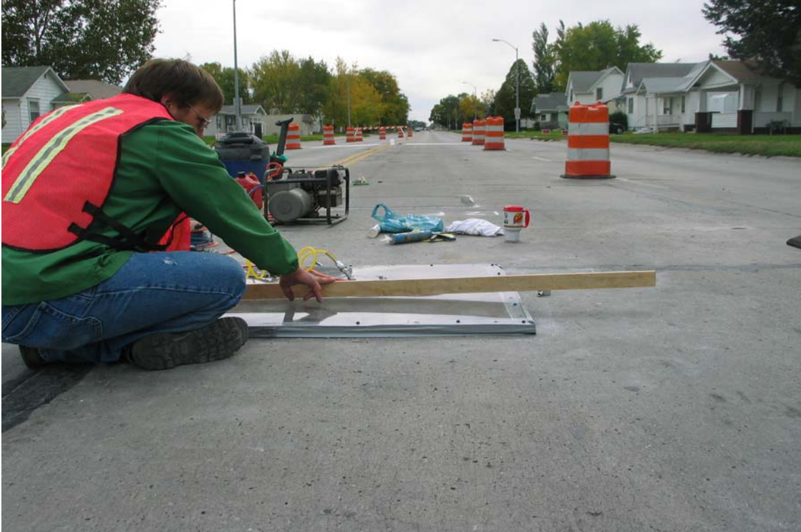
Photo No. 15 - Pressure Cell
