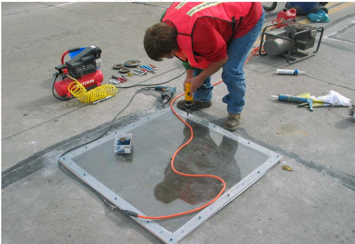
Photo No. 12 – Pressure Cell
