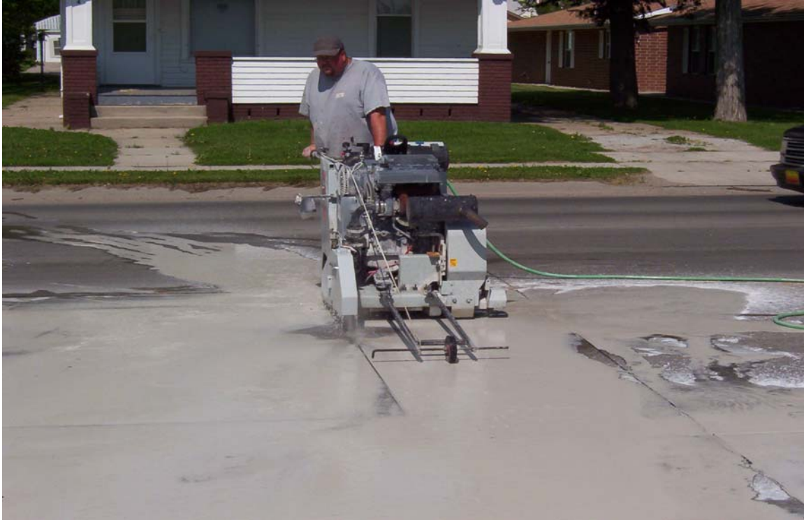
Photo No. 3 - Saw Cutting Operation
