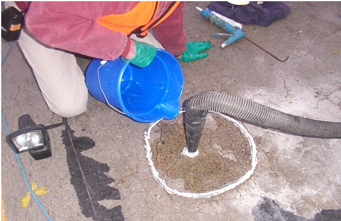
Photo No. 17 - Vacuum Impregnation of Lithium Nitrate
