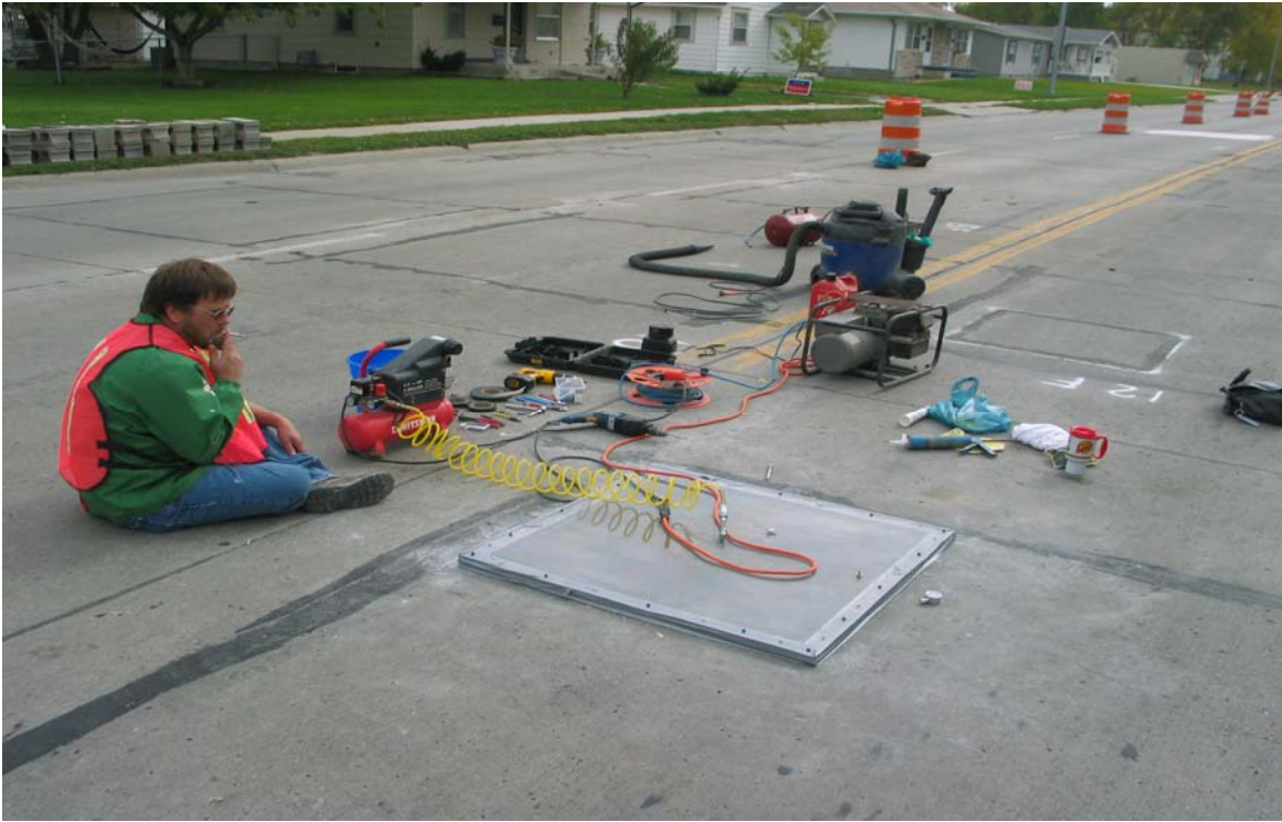
Photo No. 14 – Pressure Cell
