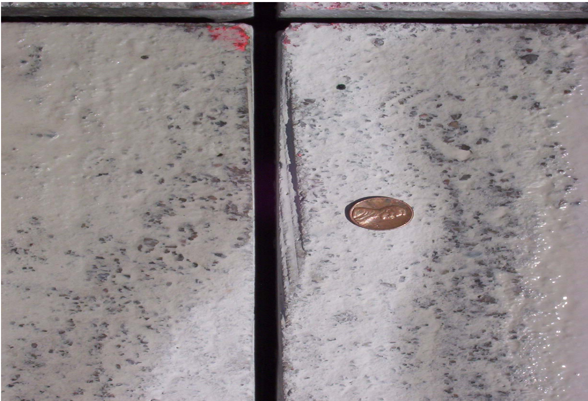
Photo No. 4 - Finished Saw Cut
