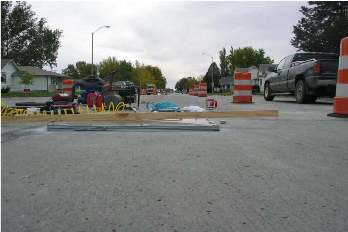
Photo No. 16 – Pressure Cell
