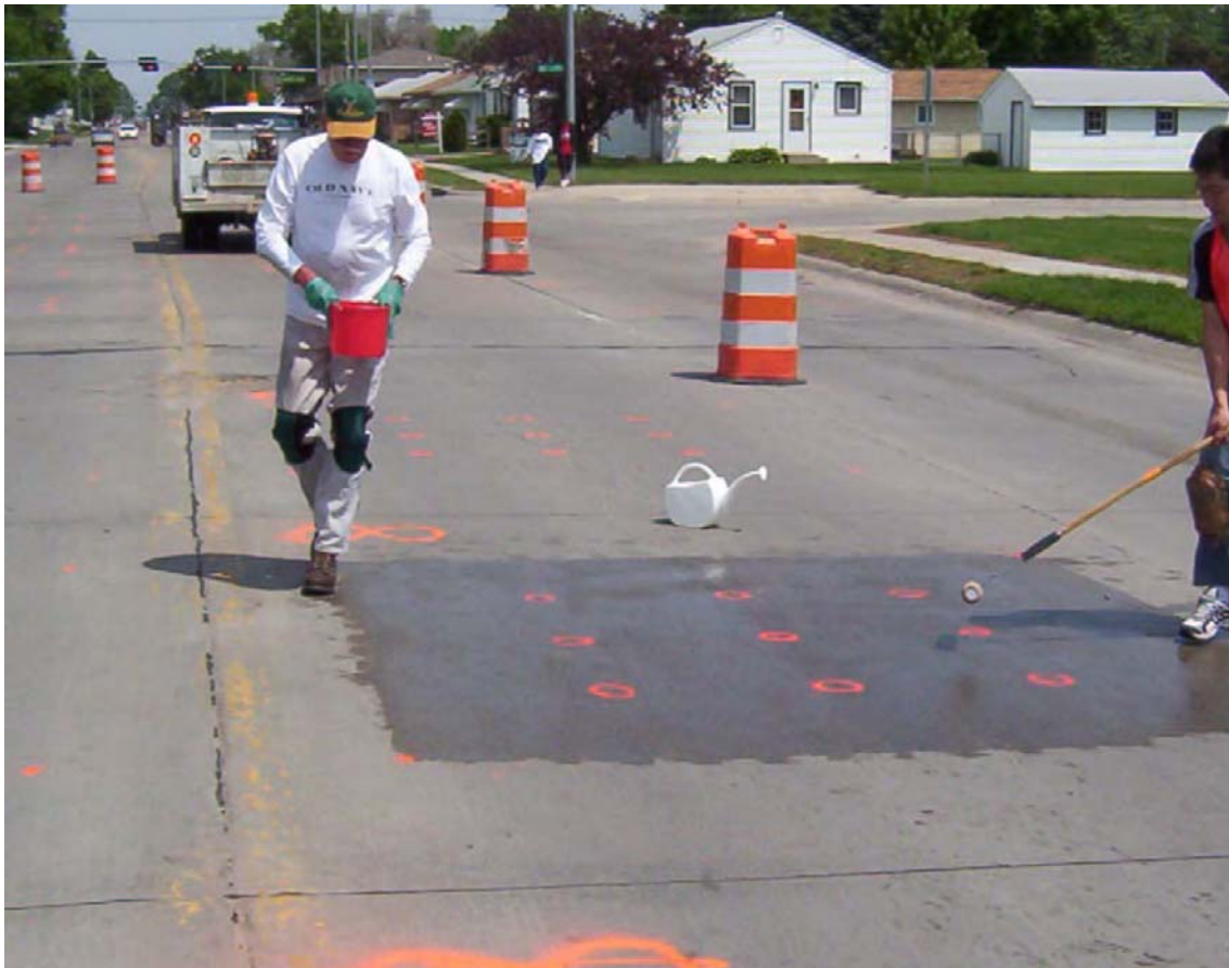
Photo No. 10 – Application of Water.
