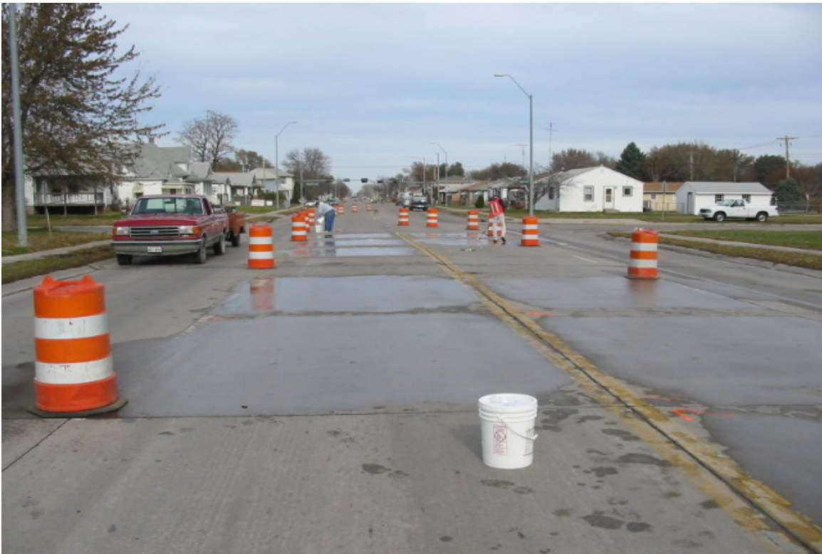
Photo No. 6 - Lithium Application
