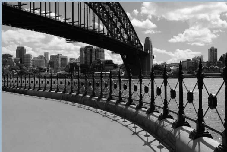
Sydney Harbour Bridge, Sydney, Australia Photography by William North
