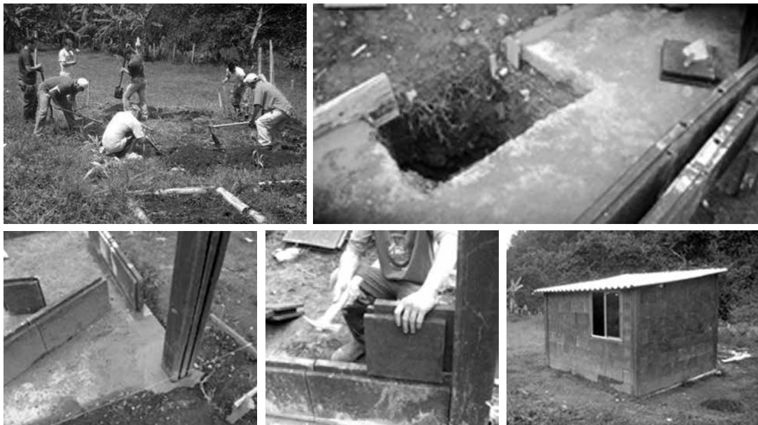
Figure 4. Ground Preparation, concrete base and columns foundations. Bricks and Columns Assembly. Finished Module.
