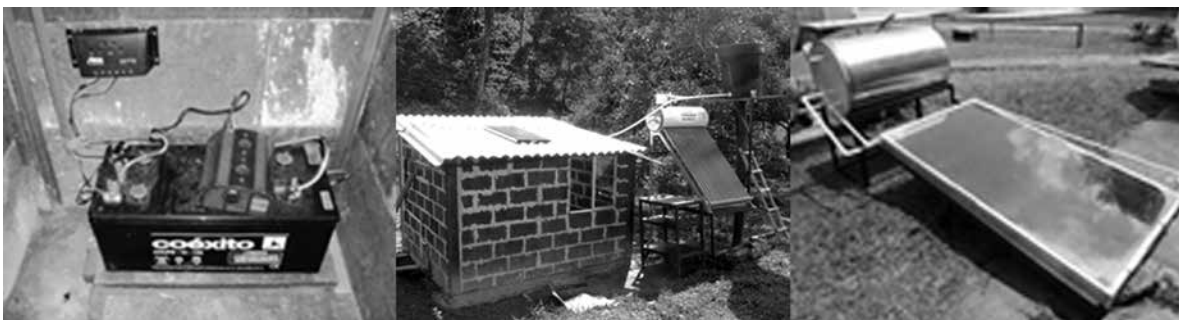
Figure 8. General and Final lay-out of the sustainable module housing: solar collector with vacuum tubes for 150 L, Photovoltaic System for 600Wh/day (20 A charge controller; 400 W Power Inverter; 100 Ah battery) and flat plate solar collector
