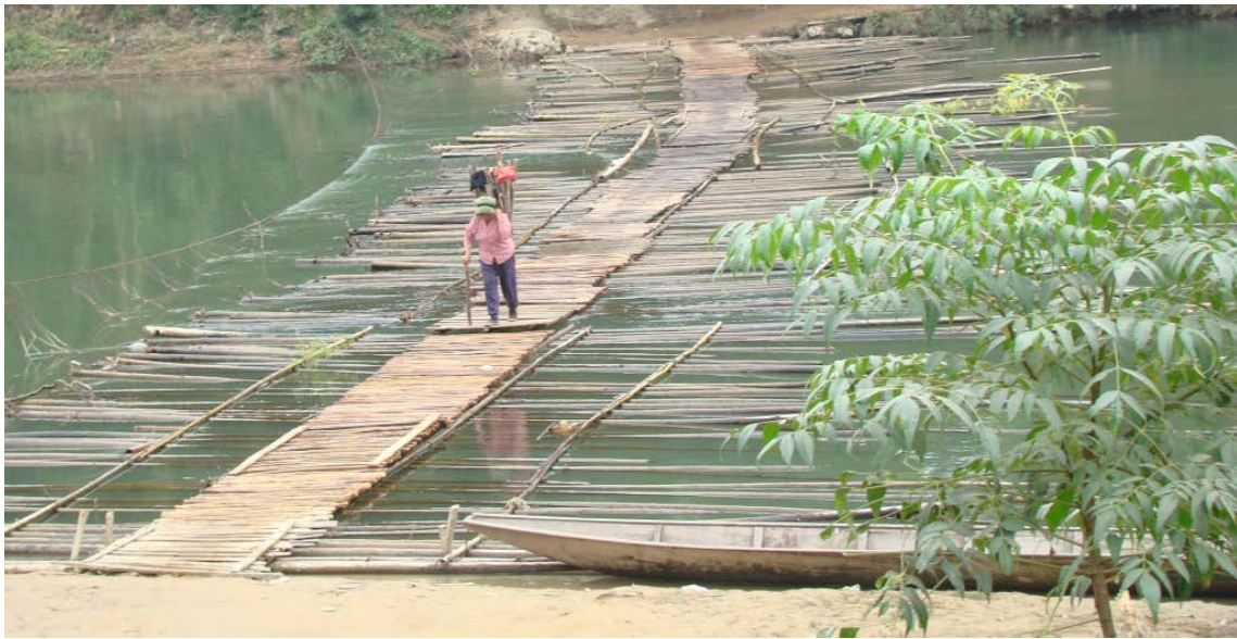
Figure 56: Some special forms of using water and possibility of floating, which could not be understood as navigation, but is in any way important for migration. These can also be the matter of different kind of early floating bridges. Bamboo floating bridge on River Xam near Xam Tai in jungle of Nam Xam Nature Reserve in western Houaphon in Laos (Photography: Josh Hirschstein ©Travel Ventures [On line] Available at: < http://hilltribeart.com/wordpress/?p=406 > [29. May 2015]).
