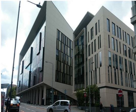
a) Outlook of the site building at University of Strathclyde.
