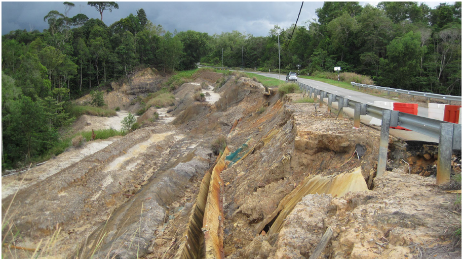
Fig. 2 An illustration of the severity of erosion process, if soil is not protected from rainfall. Labi Road, Brunei Darussalam. Photo: K. Becek
