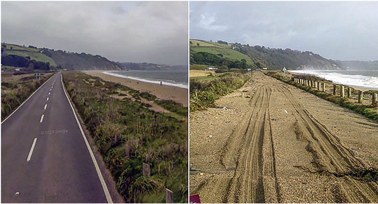
Fig. 5. Example of overwash at Slapton Sands. The road that runs along the gravel barrier of Slapton Sands, south Devon, became covered with gravel due to overwash occurring during the significant storm ‘Petra’ on 5 February 2014, but also the ‘Valentine’s Day’ storm on 14 February 2014 ( http://www.bbc.co.uk/news/uk-26064424 ).
